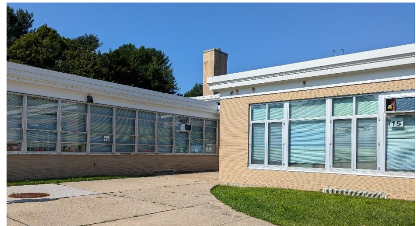
Storefront glazing utilized during the 1996 improvements project at the right of the image with the older pattern storefront windows used in classrooms on the left (above).
