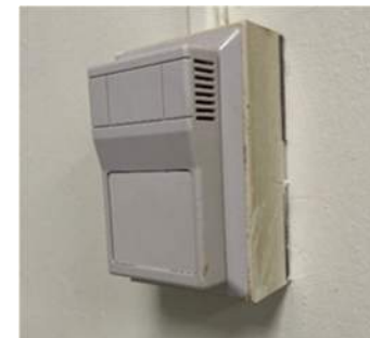
Typical BMS thermostat.
