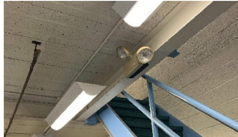
Typical self-contained battery backed emergency lighting units with twin heads in a storage space.
