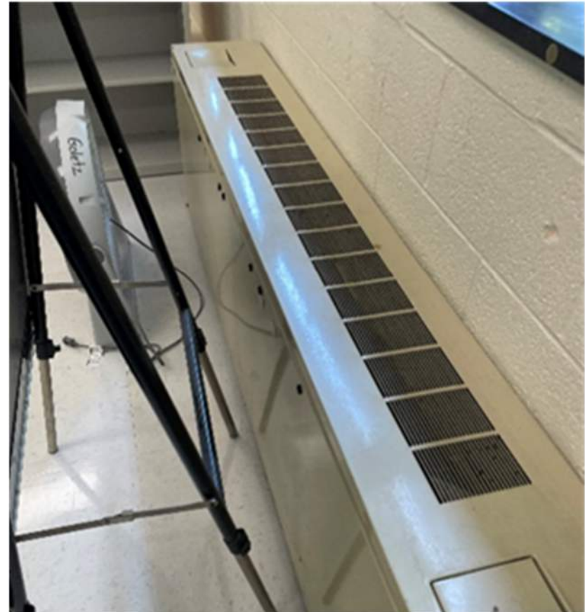
Typical perimeter unit ventilator used in classrooms.
