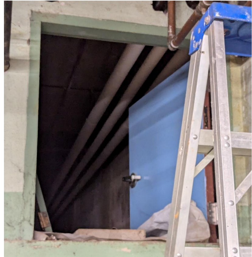
A partial height door providing access to a mechanical system crawl space that serves a portion of the original school.
