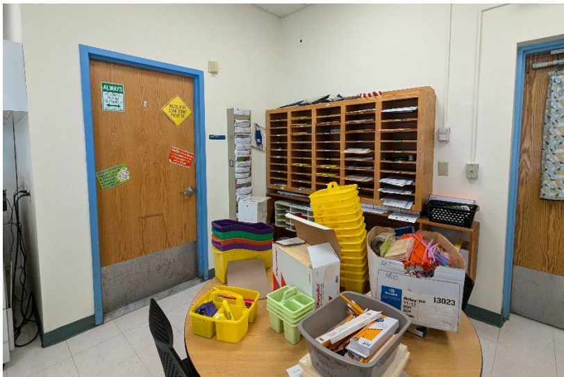
An oversized door for a single use toilet room is servicable but shows wear of its hardware and fittings.
