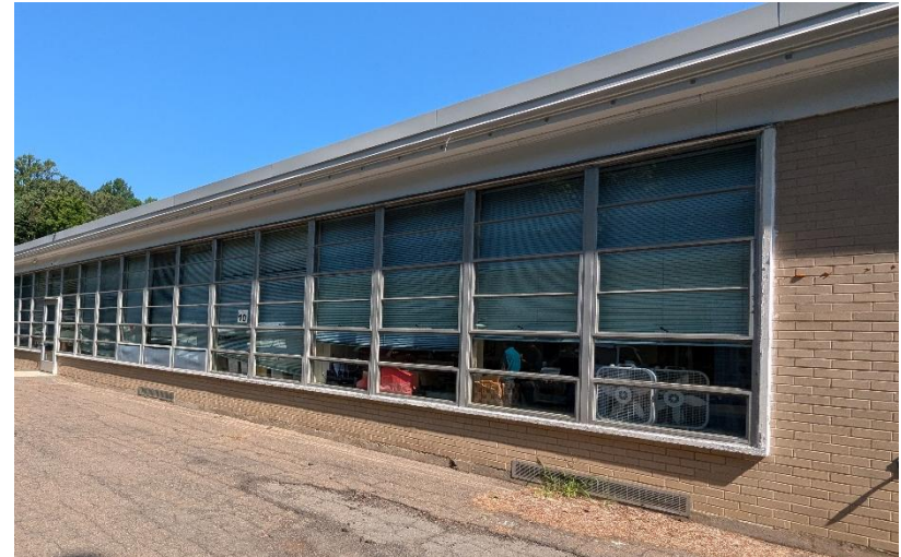
Storefront window assemblies used at pre-1996 classrooms (above)
