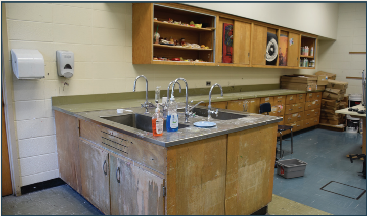
Art and science rooms are original to the construction of our buildings and are extremely outdated.
