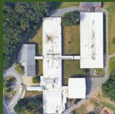
FY 26 Hood School Roof Restoration Phase II
