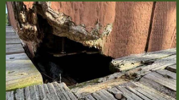
Deteriorated Exterior Trim
