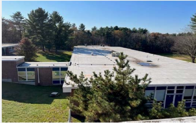
Roof Photo #17: AS is around roof top equipment and ponding water.
