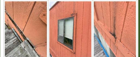
Deteriorated Exterior Trim
