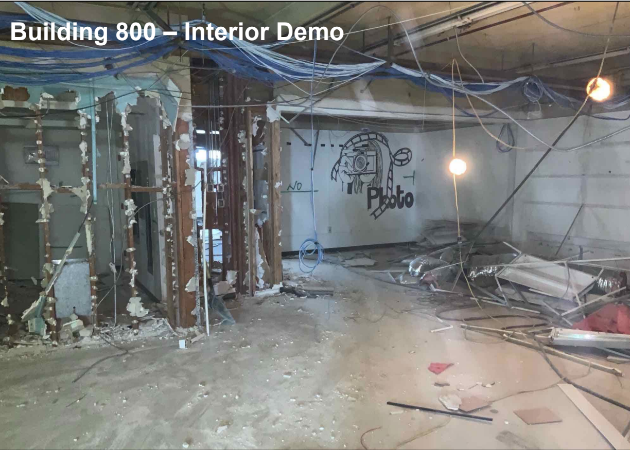
Building 800 – Interior Demo
