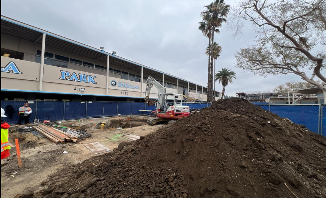
Earthwork For Foundation January 2024
