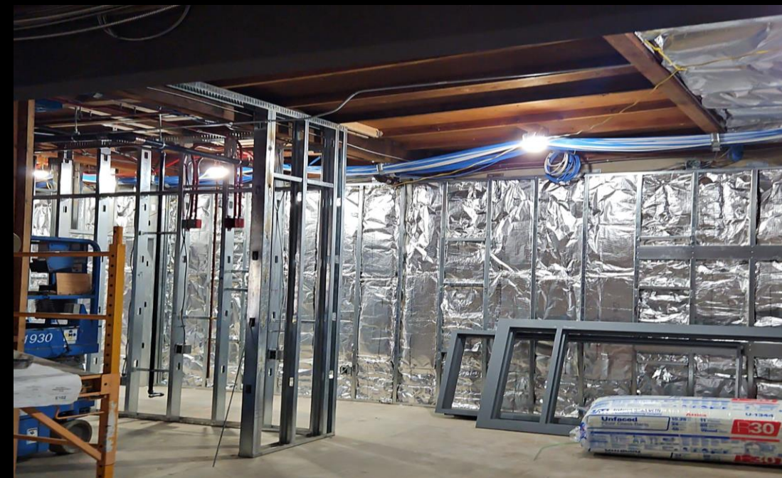
Exterior Wall Insulation January 2024
