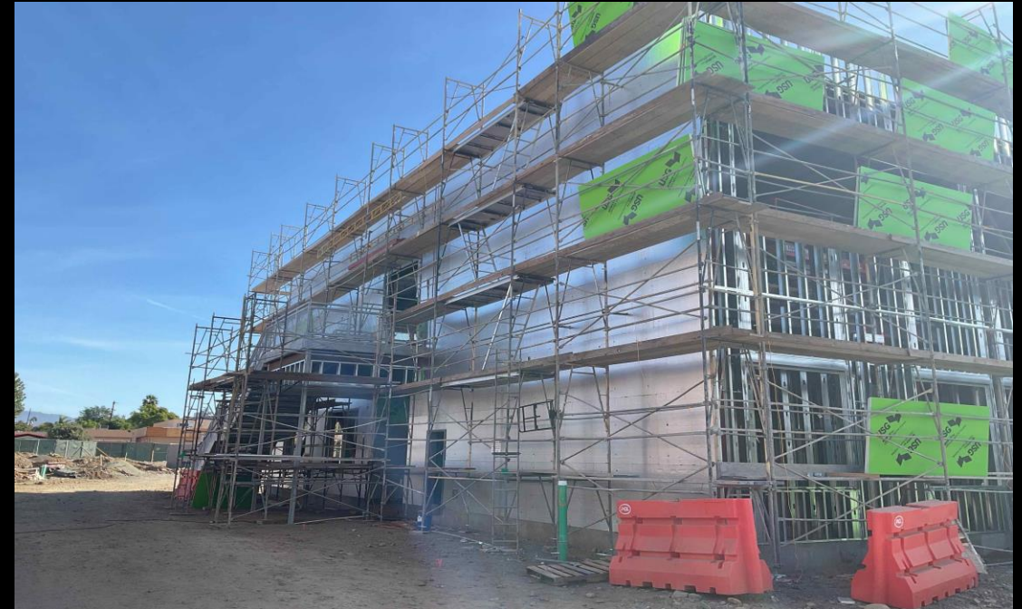
Building Envelope Closure December 2023
