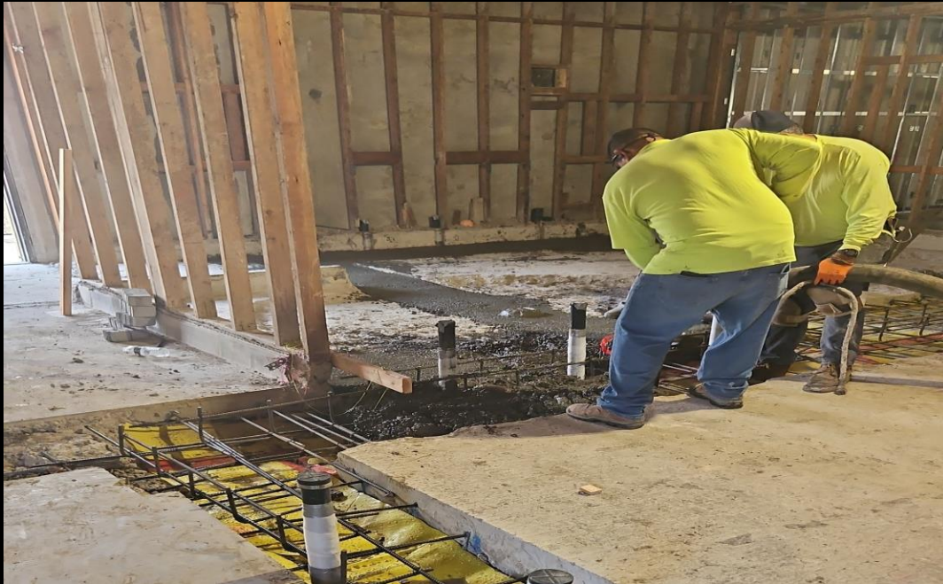
Concrete Infills September 2023
