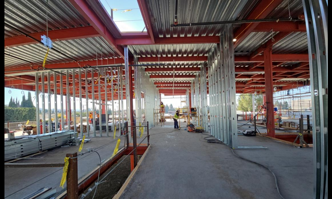
Interior Metal Framing December 2023
