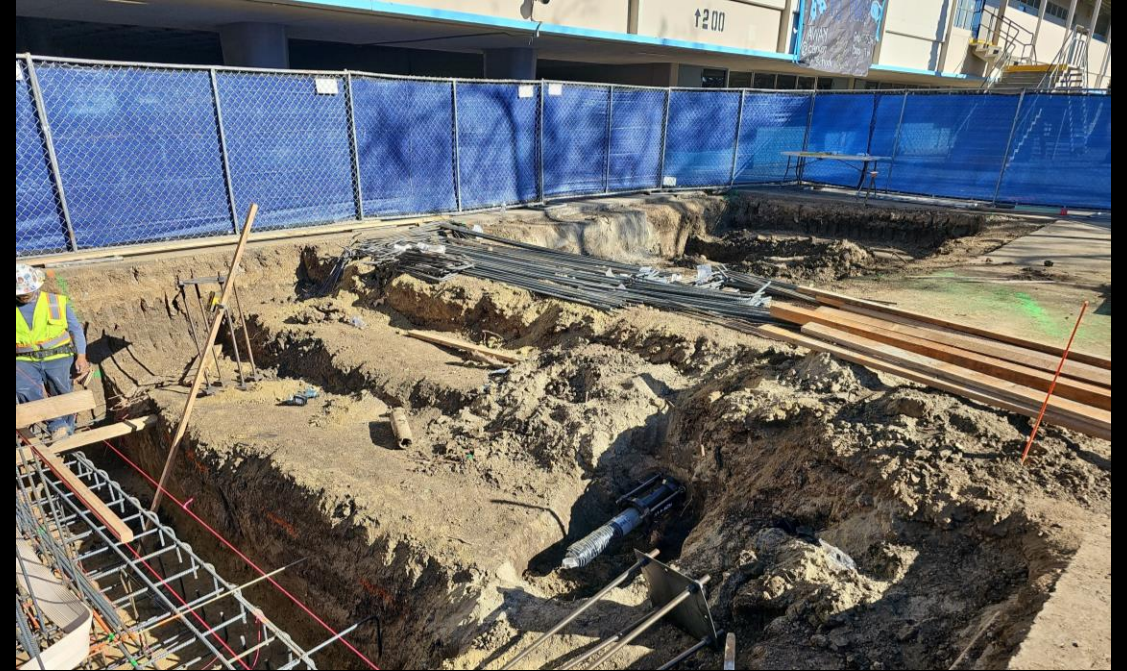
Foundation For Elevator January 2024
