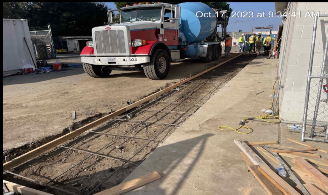
Concrete Slab Infills October 2023
