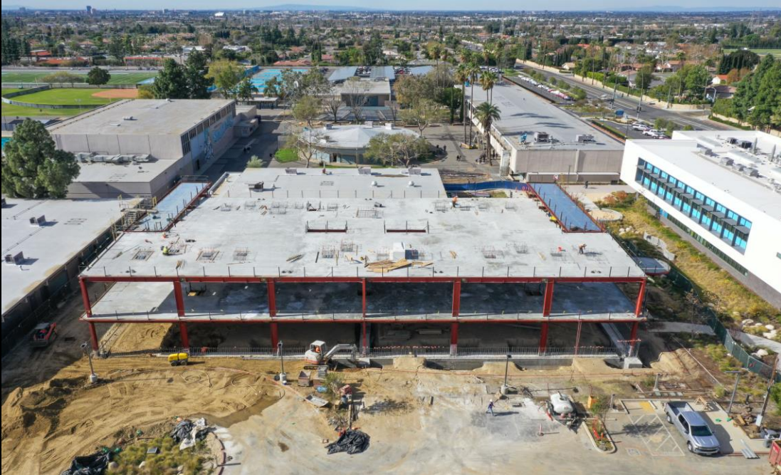
Completion of Concrete November 2023
