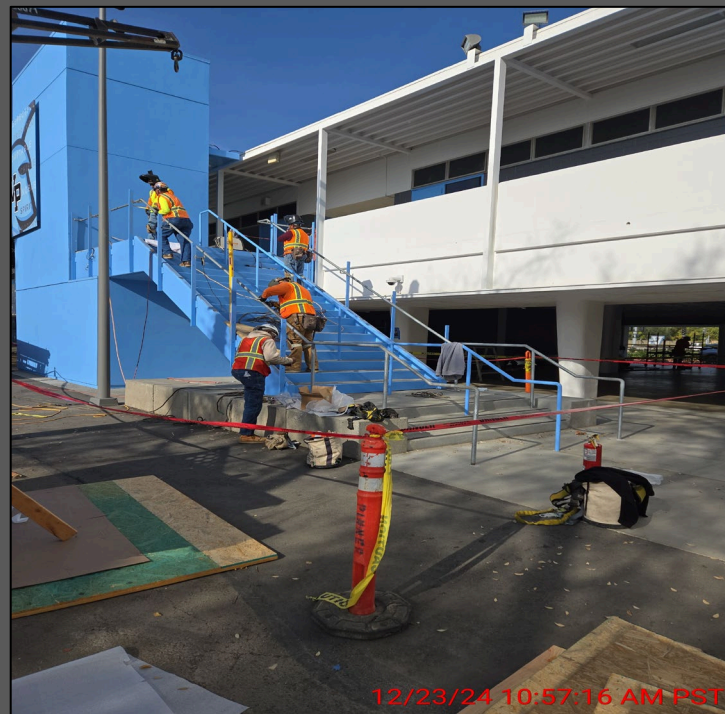
December 2024 – New Stair
