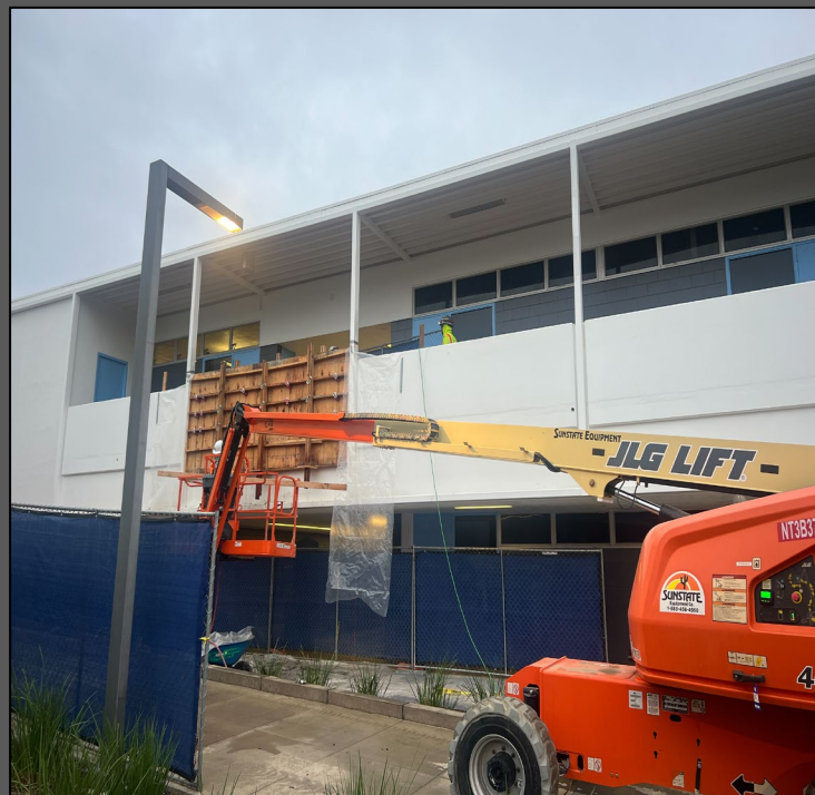
November 2024 – (E) Stair Demo.
