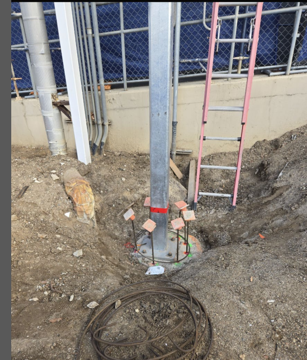
New Structural Column at Southwest Side of Building (100/200)
