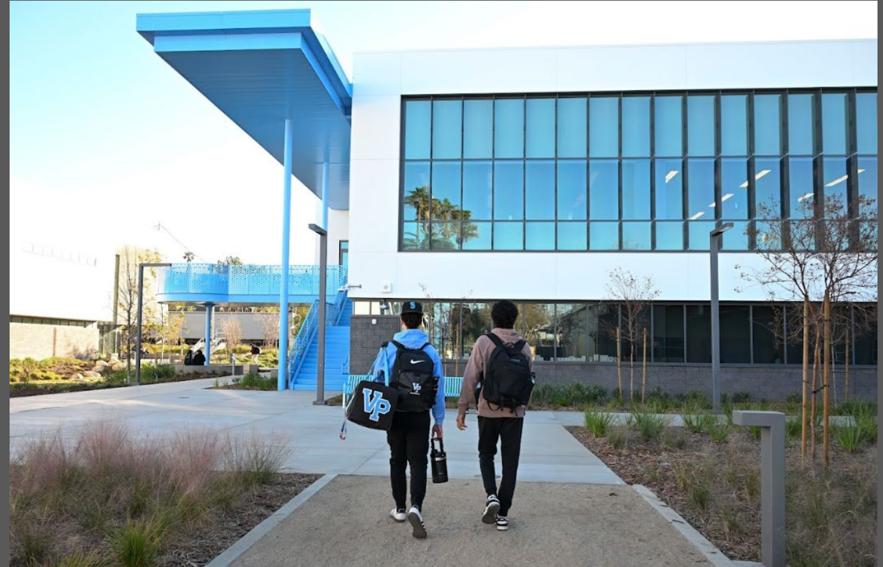
New Classroom Bldg. 500
