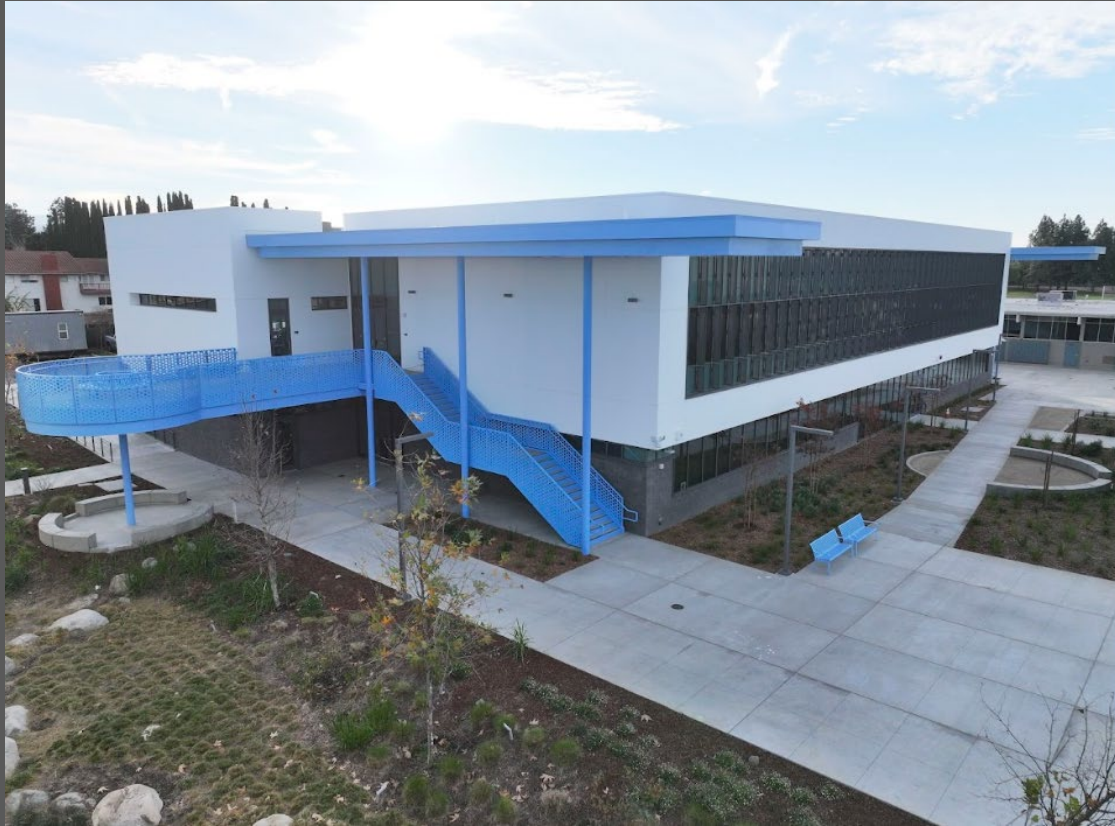
New Classroom Bldg. 500
