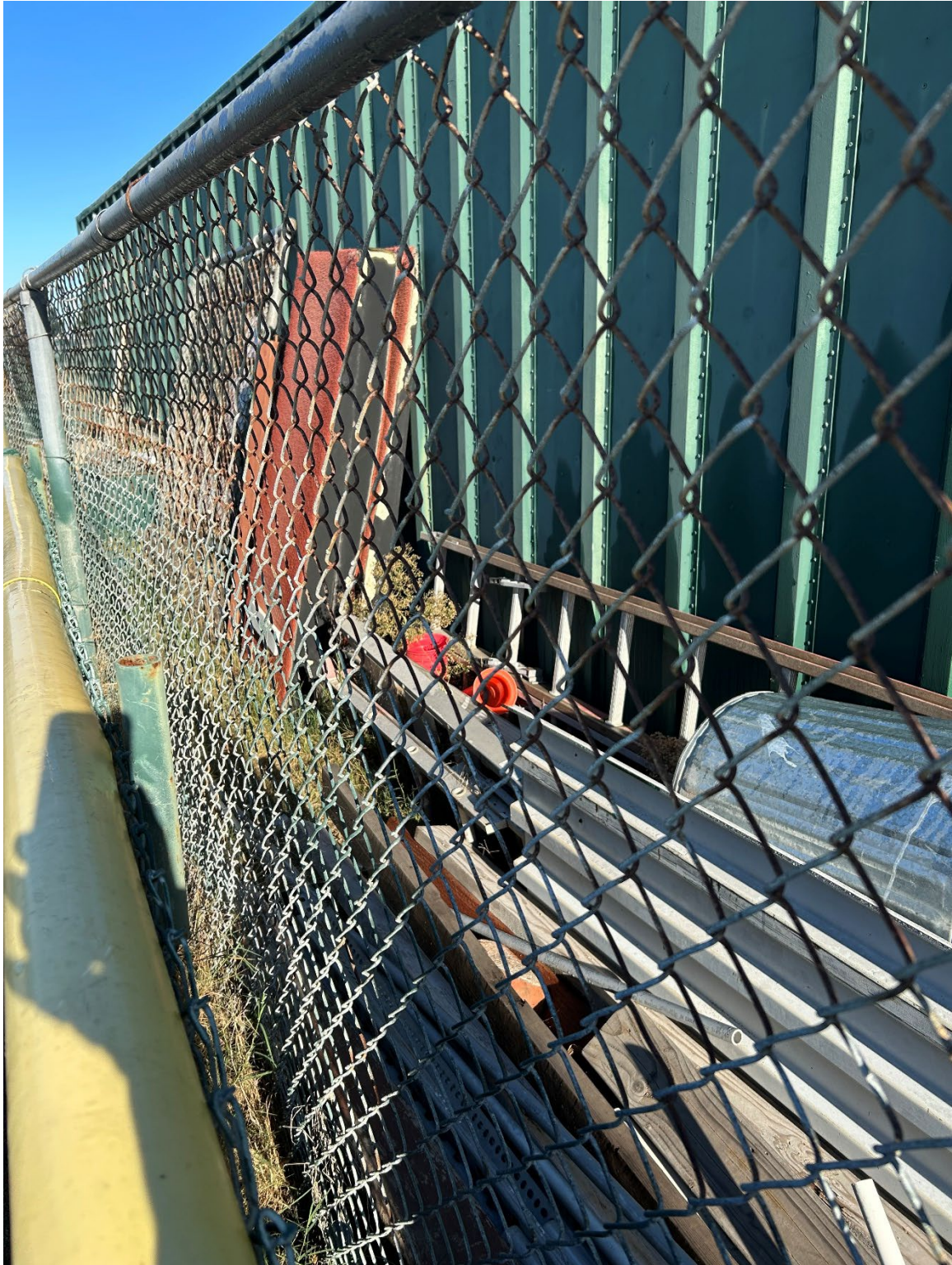
Figure 5 - Metal Pipes and Poles
