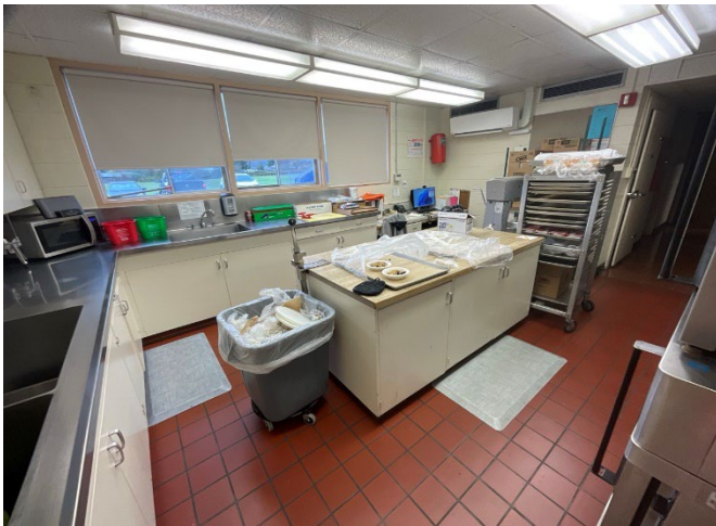
27 – COMMERCIAL KITCHEN OVERVIEW
