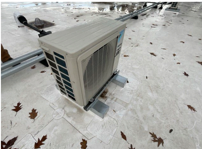
9 – SPLIT SYSTEM DUCTLESS
