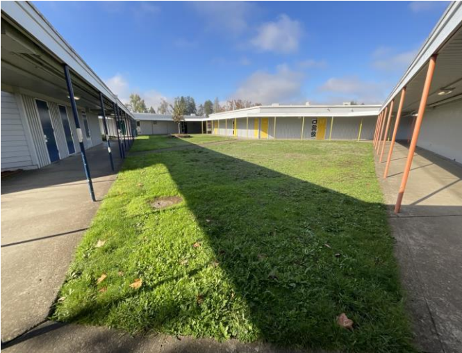
1 - EXTERIOR COVER CORRIDORS
