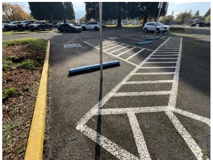
4 - ASPHALT PARKING LOTS
