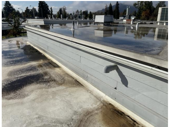
8 - PRIMARY ROOF OVERVIEW
