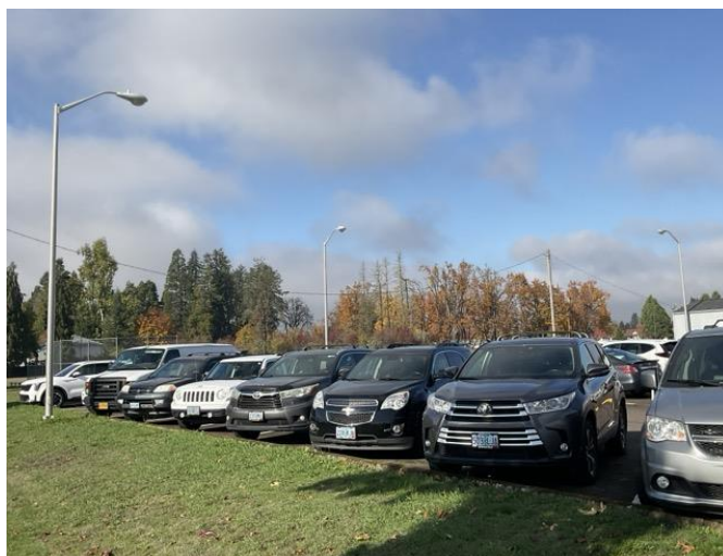
12 - POLE LIGHT FIXTURE WITH LAMPS
