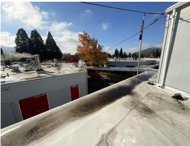
3 - PRIMARY ROOF OVERVIEW
