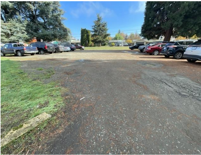
5 - GRAVEL PARKING LOT
