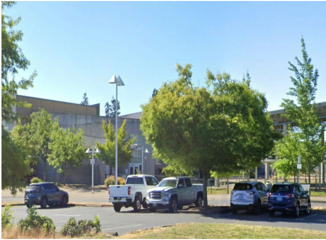
7 – EXTERIOR SITE LIGHTING
