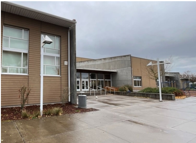
3 – EXTERIOR SITE LIGHTING
