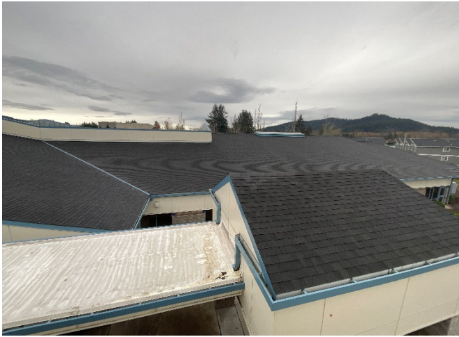
7 – PRIMARY ROOF OVERVIEW
