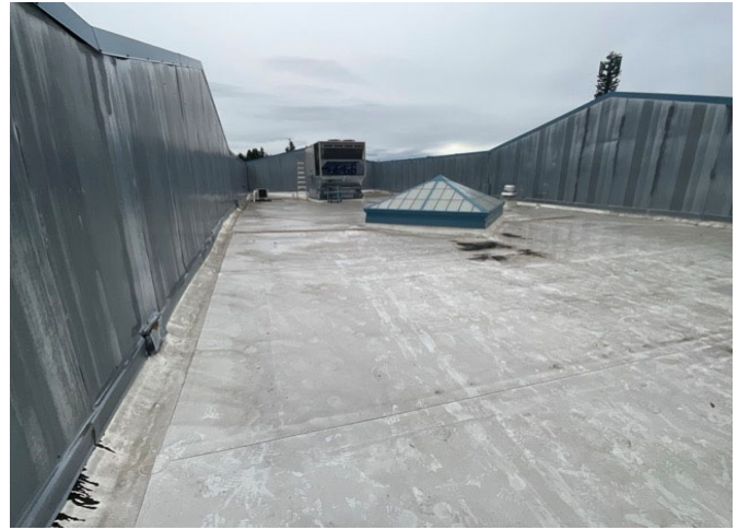
8 – SECONDARY ROOF OVERVIEW
