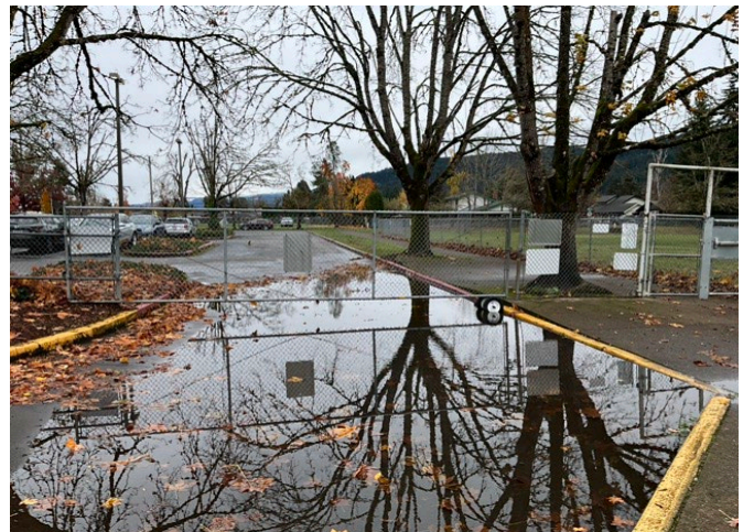
6 – PONDING IN PARKING LOT
