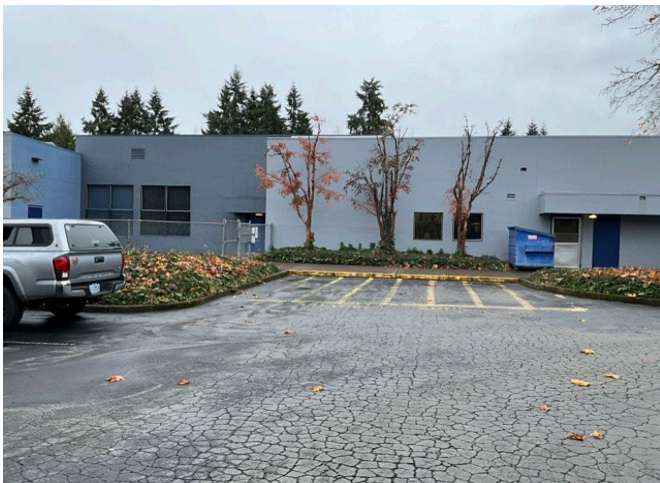
5 – PARKING LOT AREA
