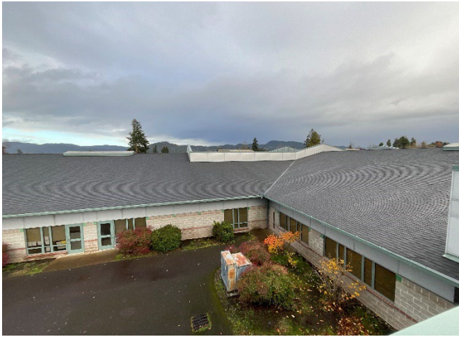
7 – PRIMARY ROOF OVERVIEW
