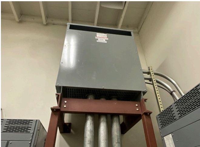
27 – SECONDARY TRANSFORMER
