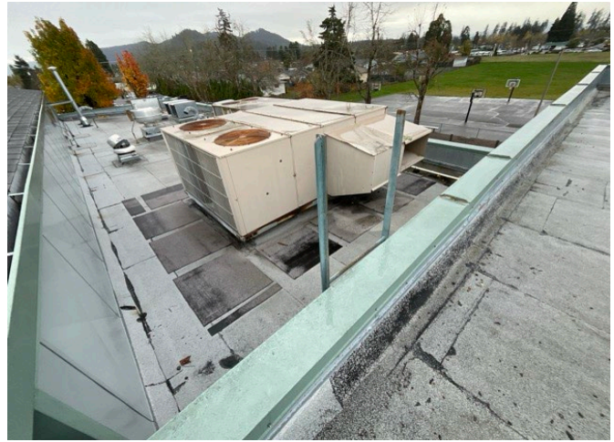
8 – SECONDARY ROOF OVERVIEW
