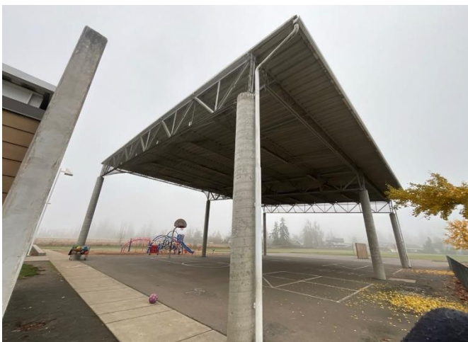
11 – COVERED PARKING STRUCTURE
