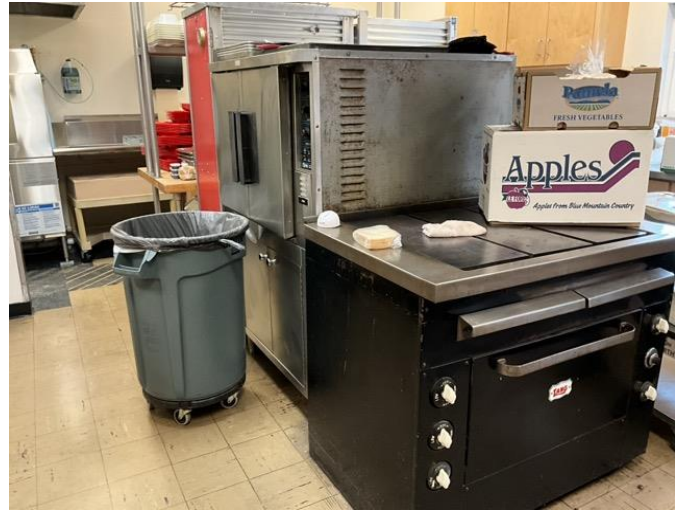
24 - COMMERCIAL KITCHEN LINE
