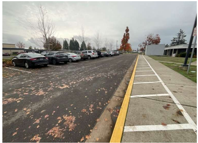
4 – MAIN PARKING LOT
