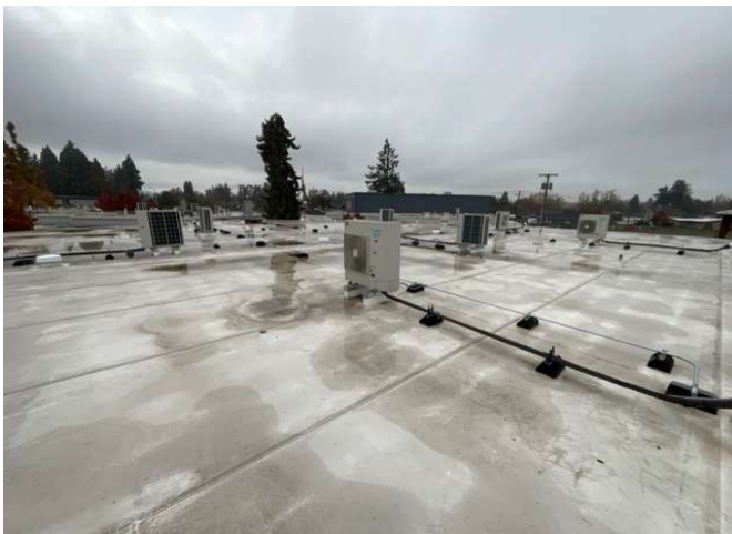
23 – PRIMARY ROOF OVERVIEW
