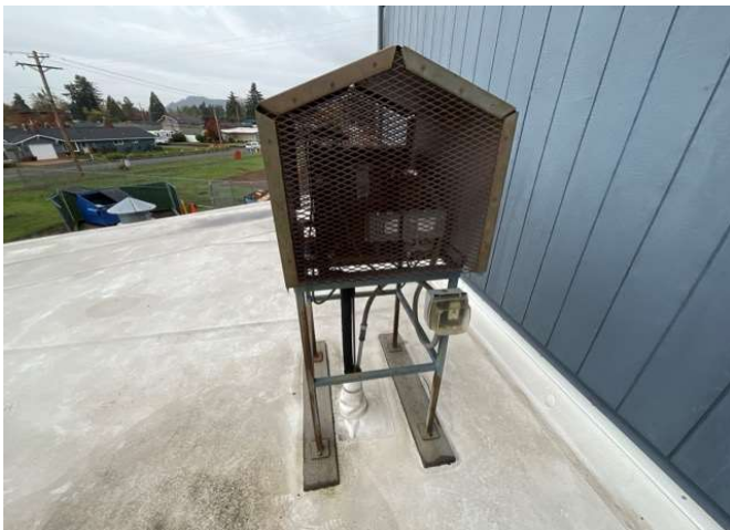
17 – CONDENSING UNIT FOR WALK-IN CO
