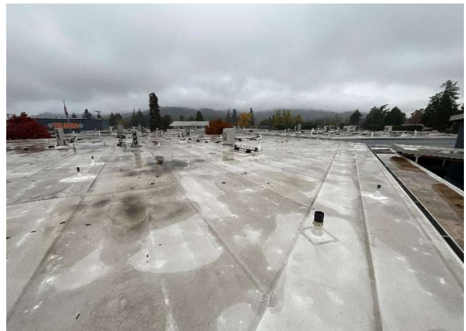
18 – PRIMARY ROOF OVERVIEW
