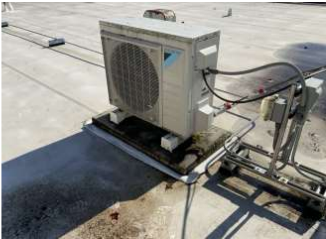
21 - SPLIT SYSTEM DUCTLESS
