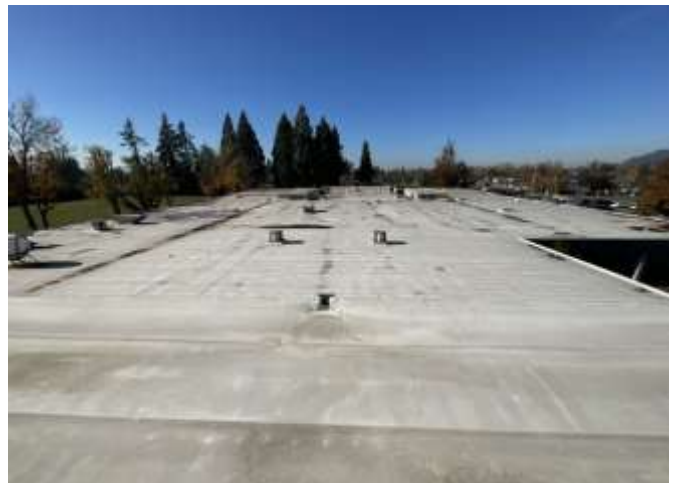
6 - PRIMARY ROOF OVERVIEW
