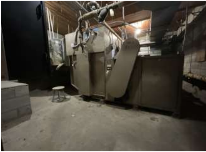
19 - AIR HANDLERS WITH DX COILS
