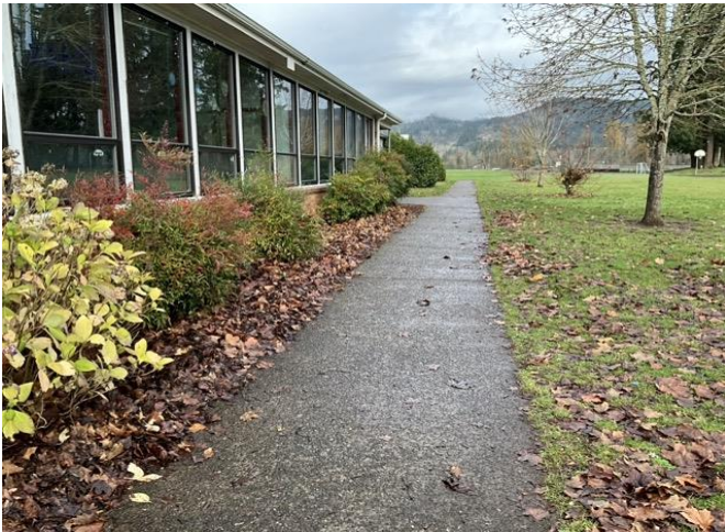
1 – LANDSCAPING AND WALKWAY
