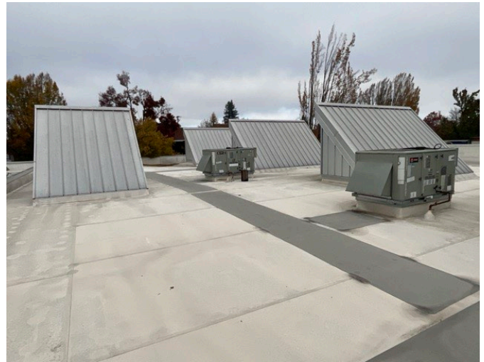
8 - SECONDARY ROOF OVERVIEW
