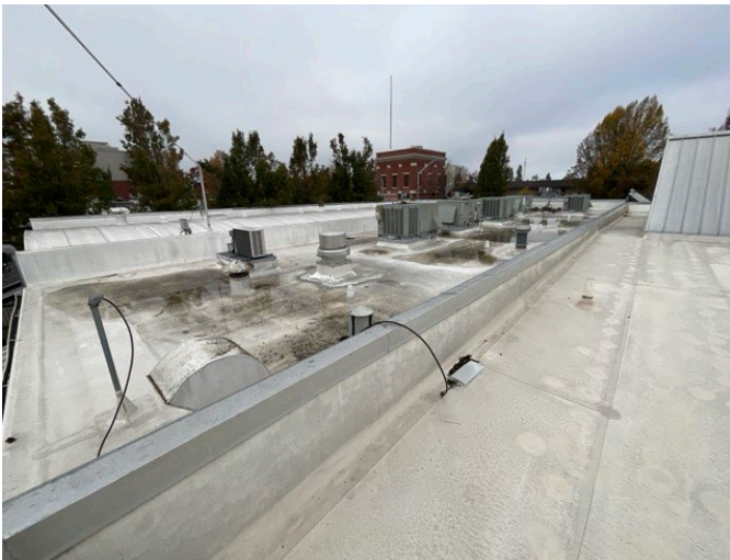
9 - PRIMARY ROOF OVERVIEW
