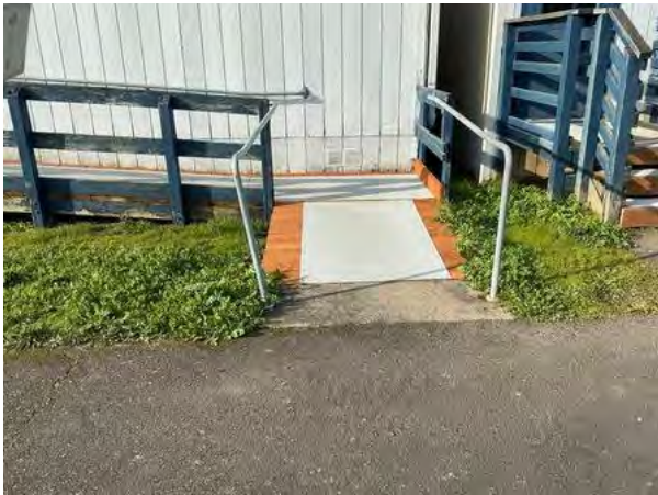
Photos for Barrier ID: AX557623
