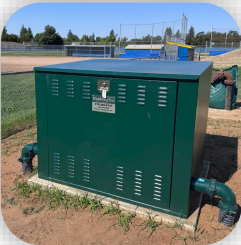
Irrigation pump replacement for sports fields at Del Campo High School
