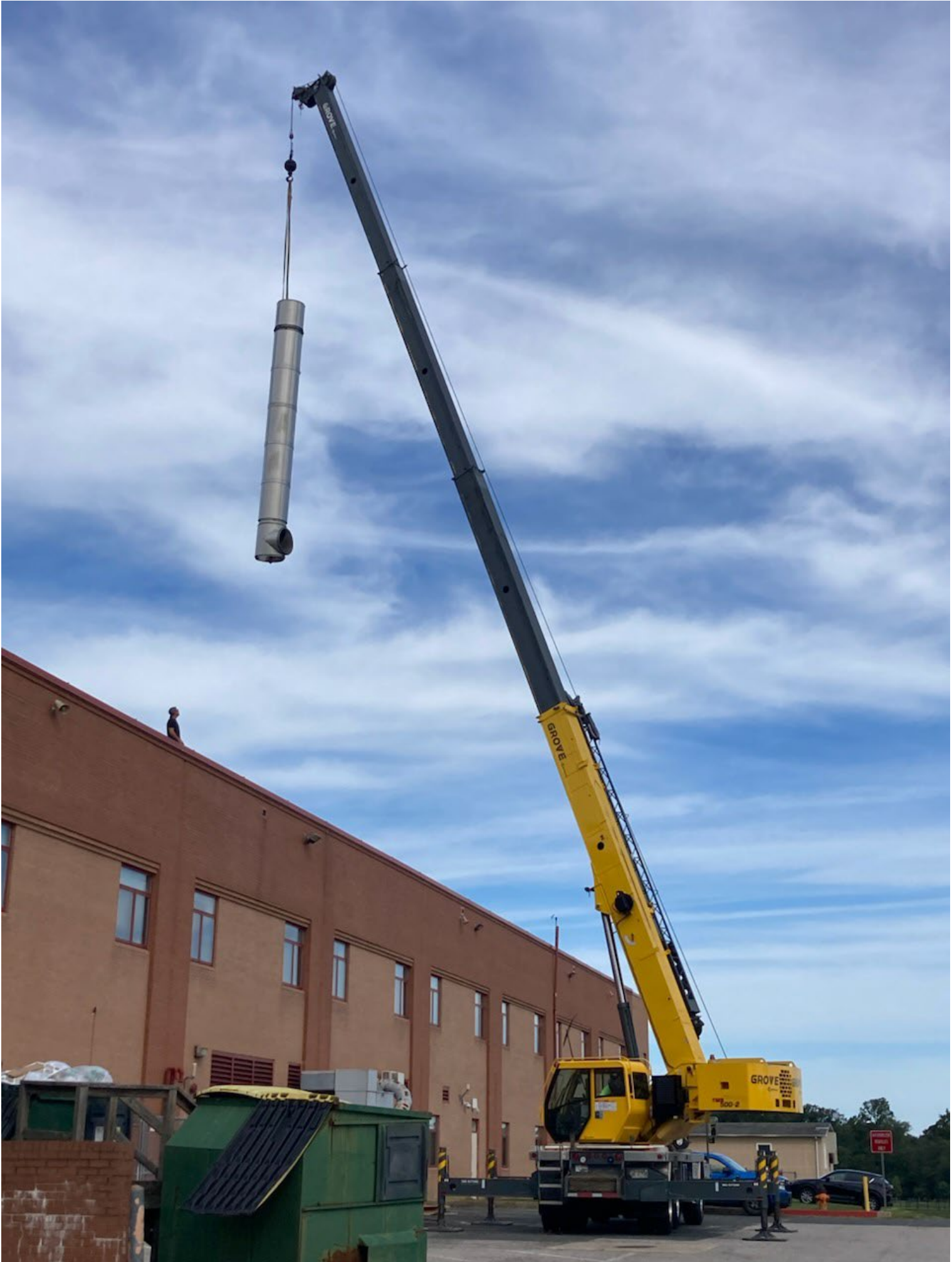
RISING SUN HIGH SCHOOL – BOILER STACK REPLACEMENT
