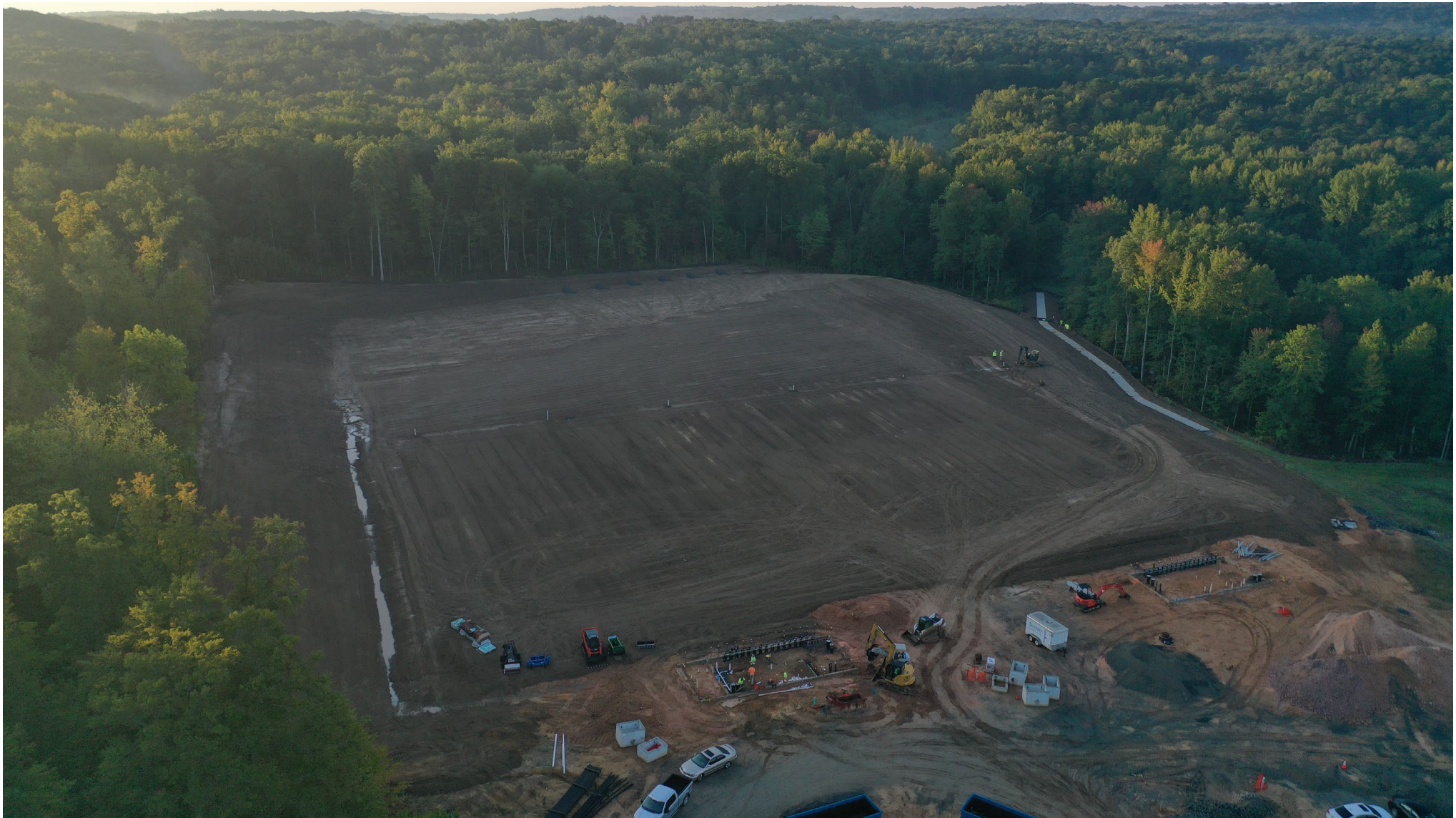
NORTH EAST MIDDLE / HIGH SCHOOL – REPLACEMENT
