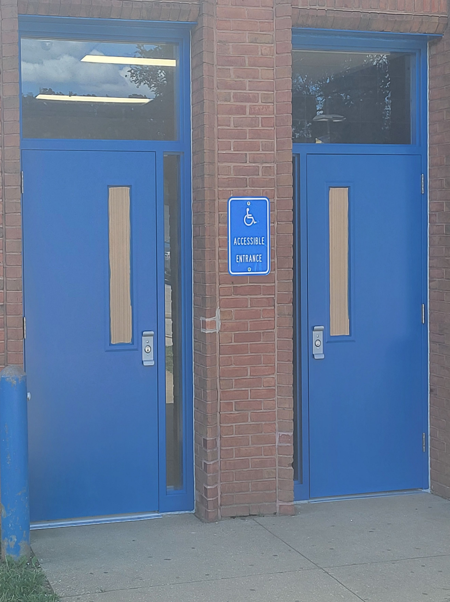
PERRYVILLE HIGH SCHOOL – EXTERIOR DOORS REPLACEMENT
