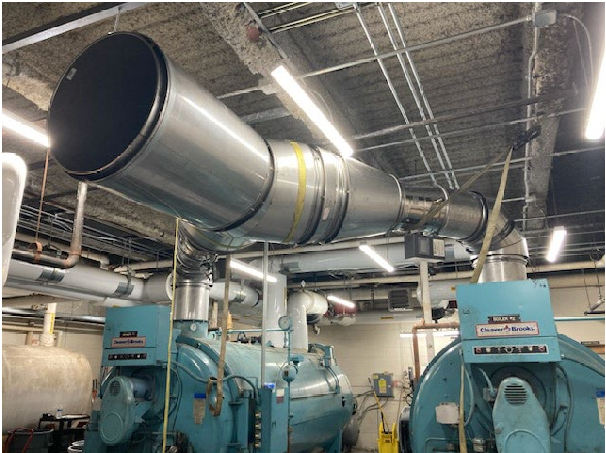
RIISING SUN HIGH SCHOOL – BOILER STACK REPLACEMENT
