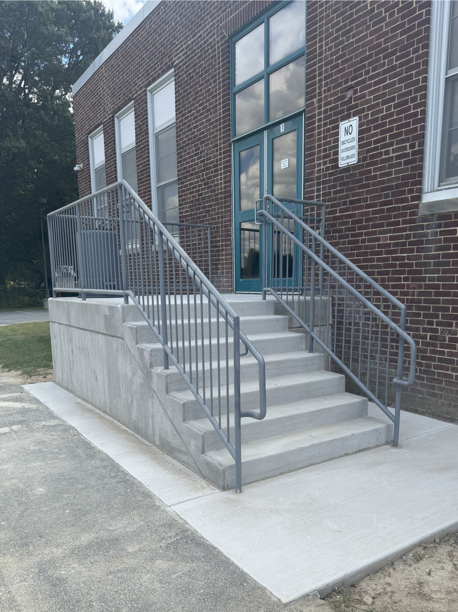
CECILTON ELEMENTARY SCHOOL – EXTERIOR STEPS REPLACEMENT
