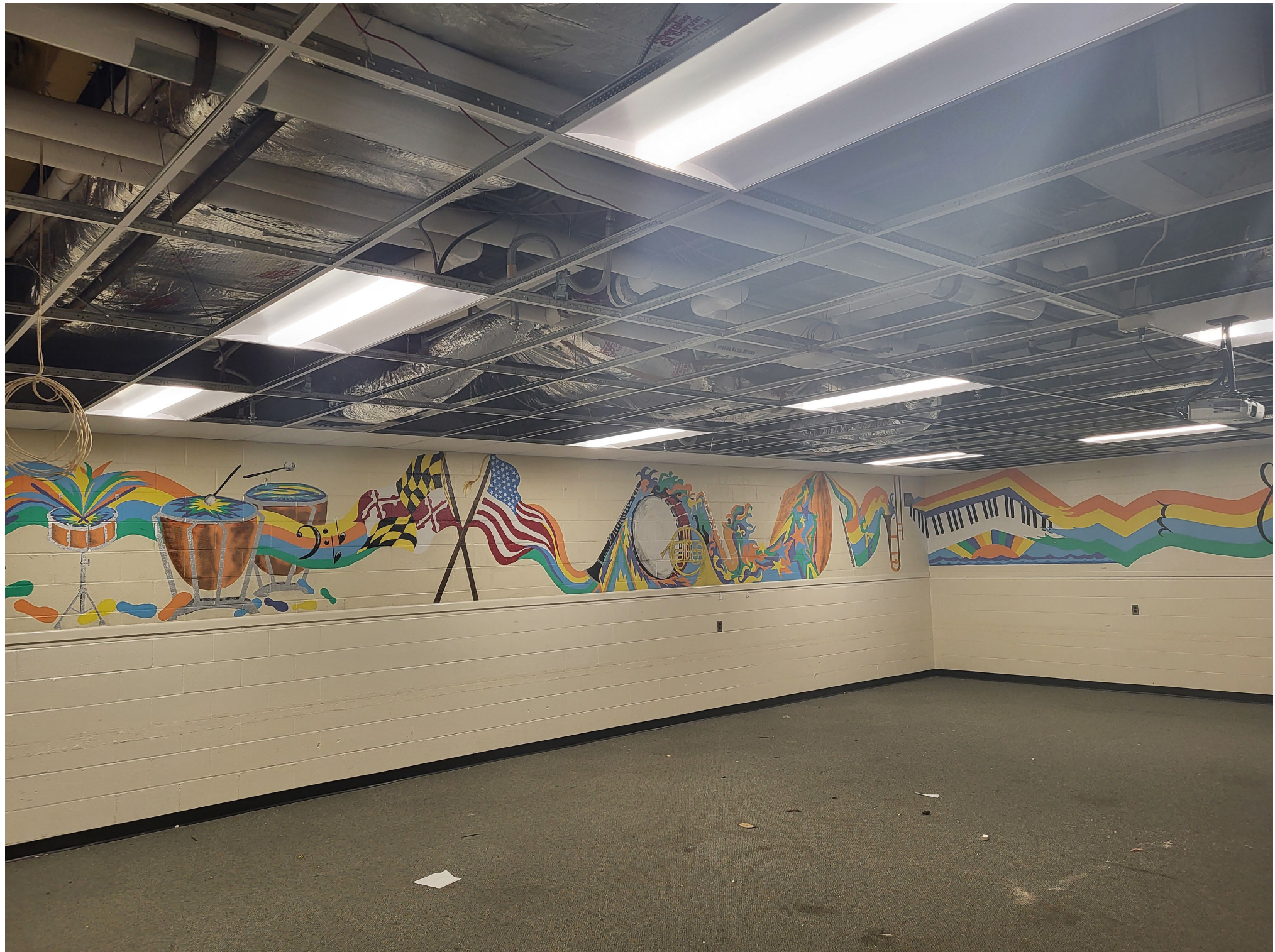
CHERRY HILL MIDDLE SCHOOL – PIPE INSULATION & CEILING REPLACEMENT
