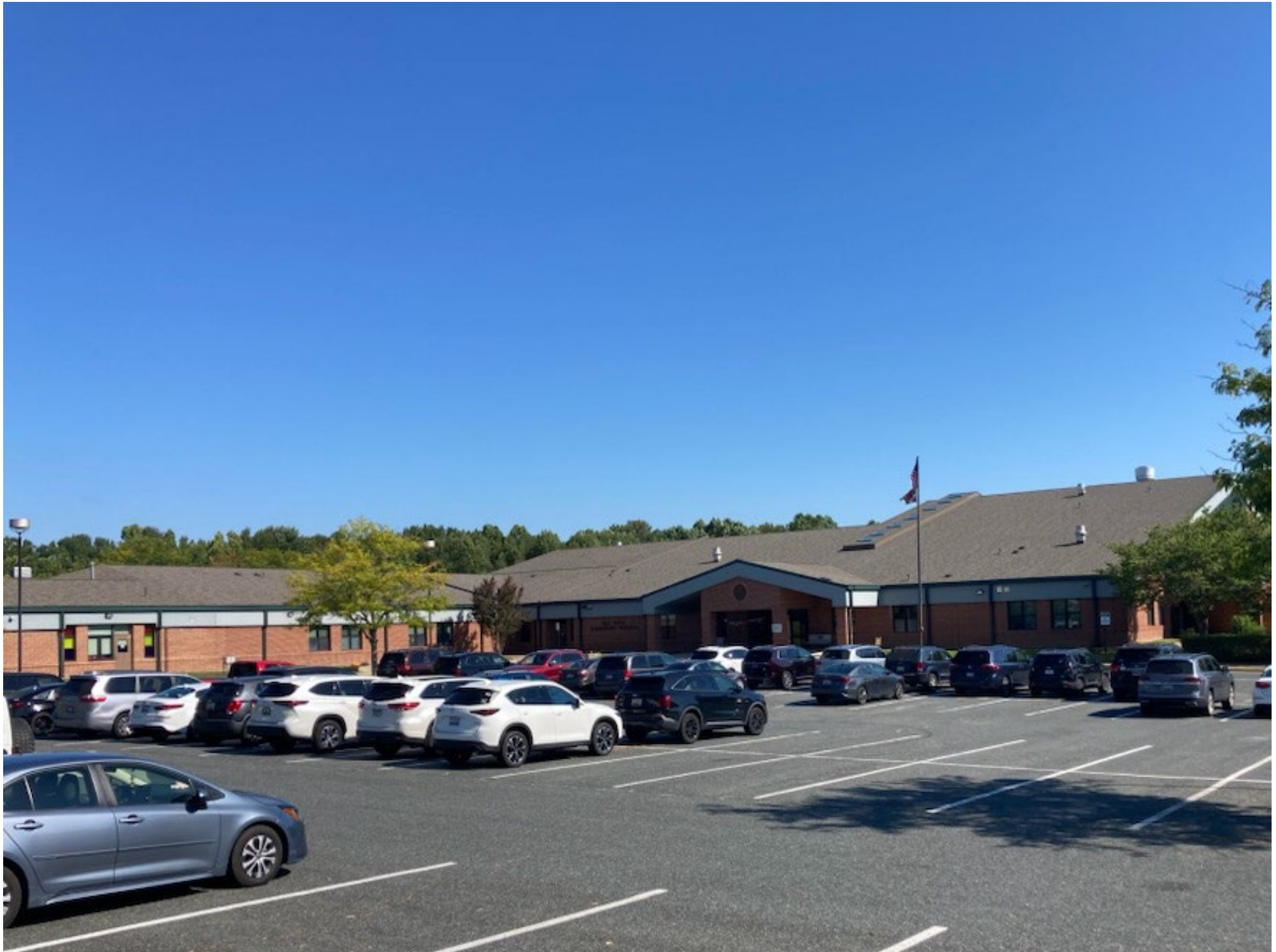
ELK NECK ELEMENTARY SCHOOL – ROOF REPLACEMENT
