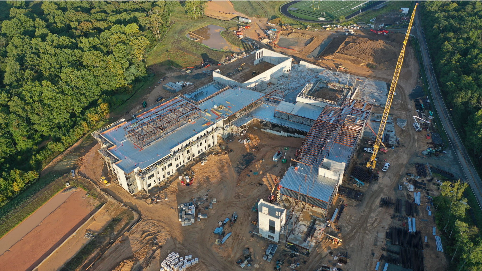
NORTH EAST MIDDLE / HIGH SCHOOL – REPLACEMENT
