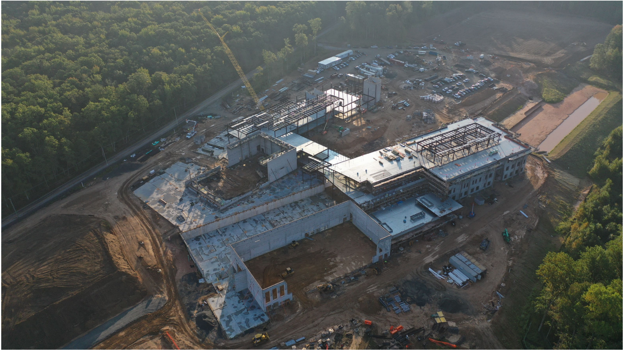
NORTH EAST MIDDLE / HIGH SCHOOL – REPLACEMENT
