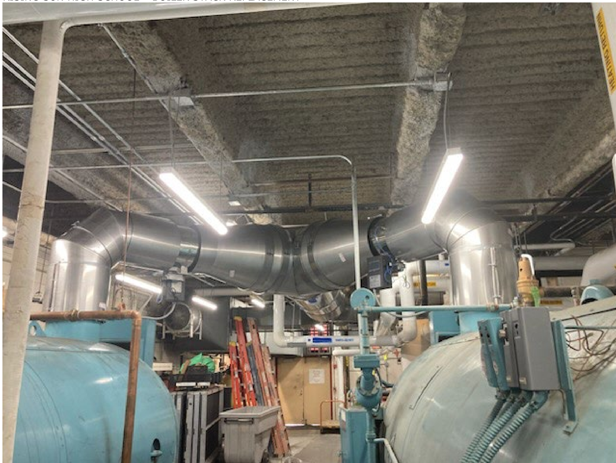
RIISING SUN HIGH SCHOOL – BOILER STACK REPLACEMENT
