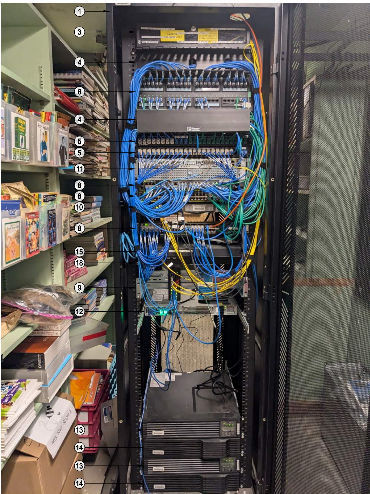
RACK - EXISTING CONDITION
