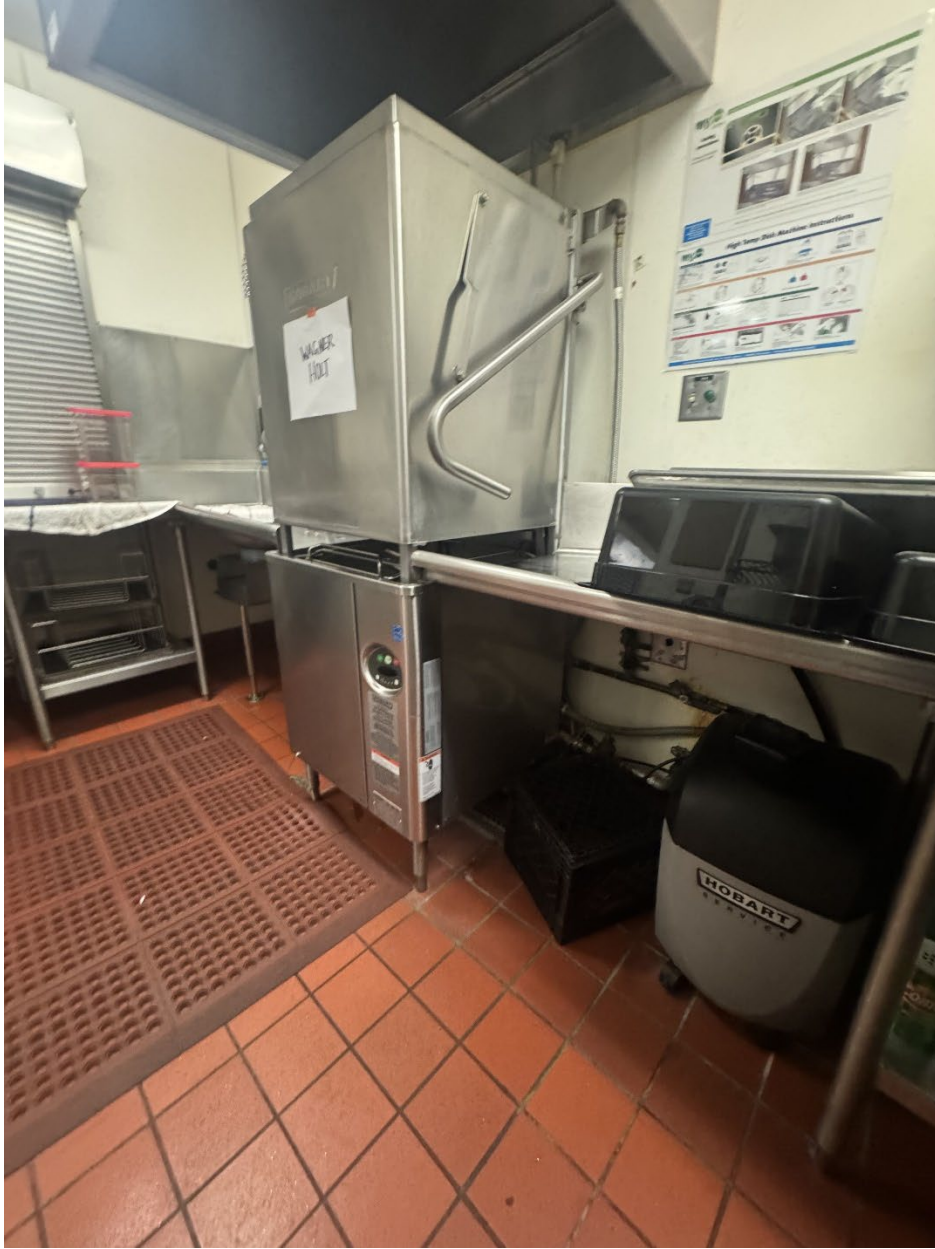
Wagner Holt Elementary School
