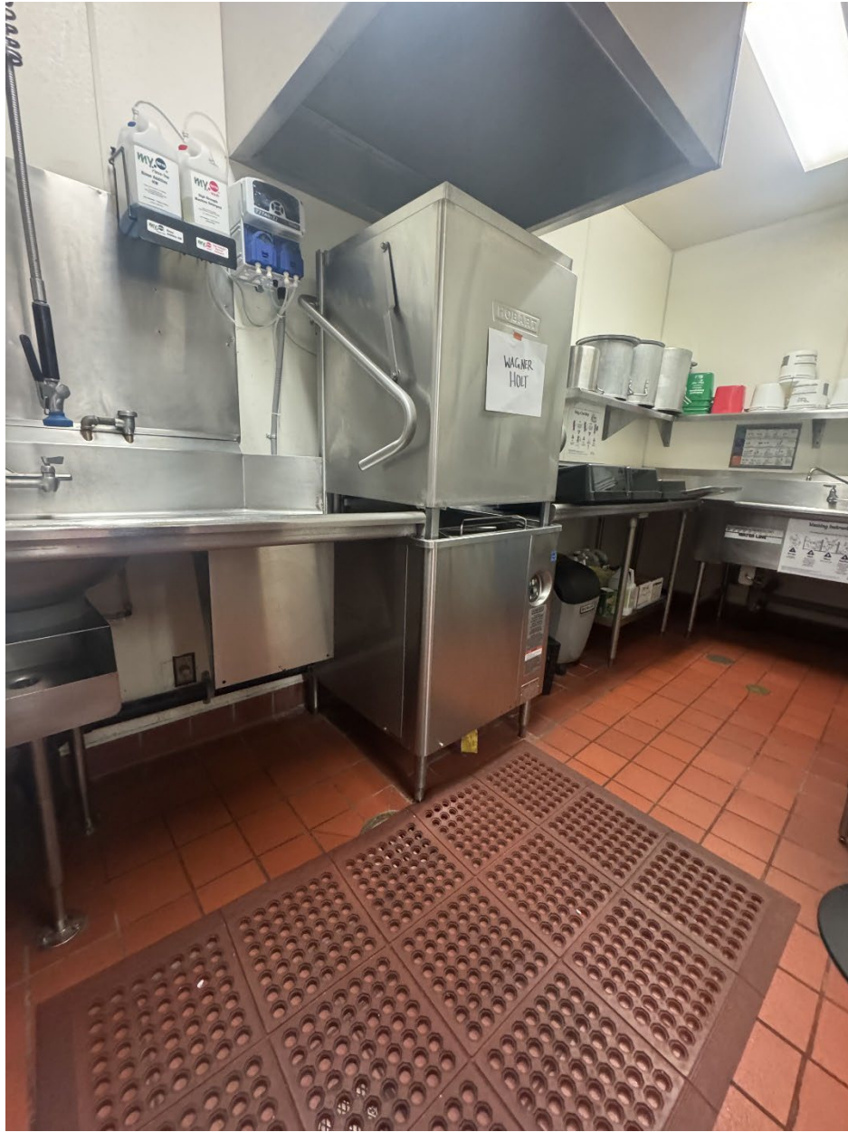
Wagner Holt Elementary School
