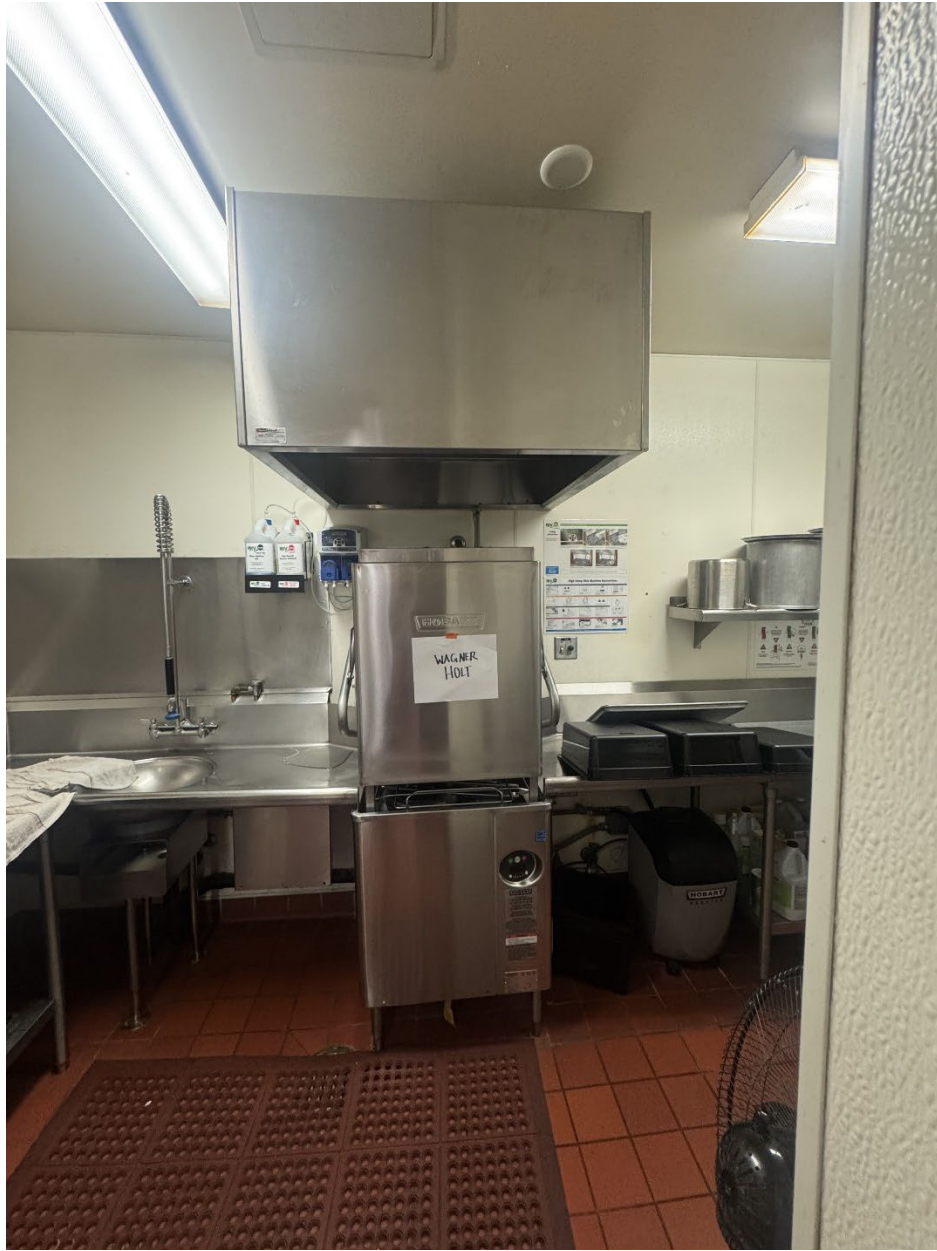
Wagner Holt Elementary School
