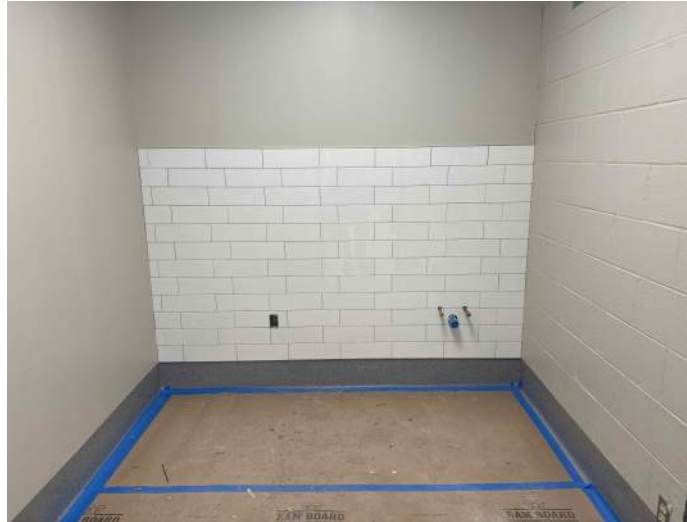
Restroom/Changing room wall tile
