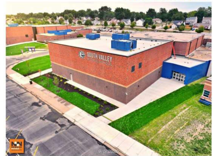
SVMS Exterior View
