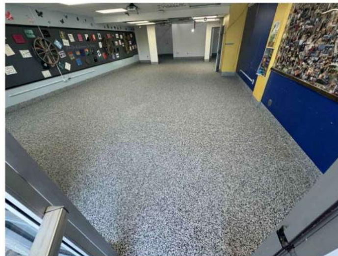
PR08 Epoxy Flooring Complete
