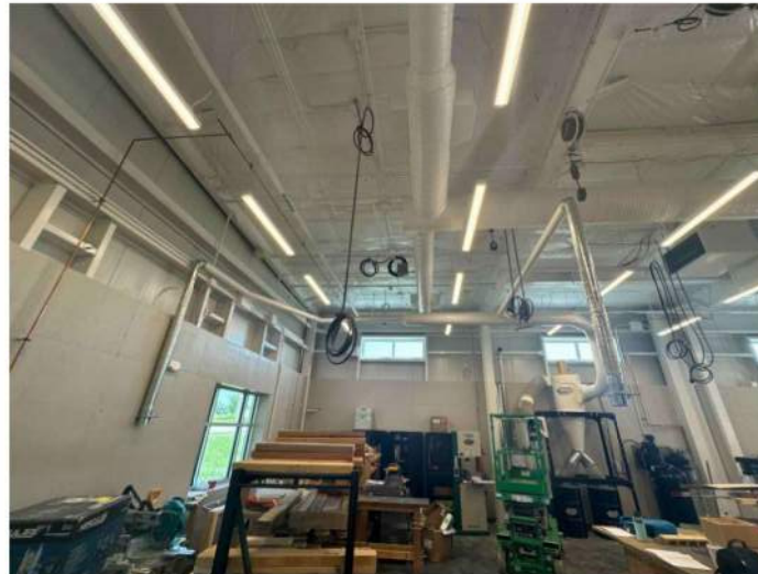
Dust Collection Install Complete in Shop
