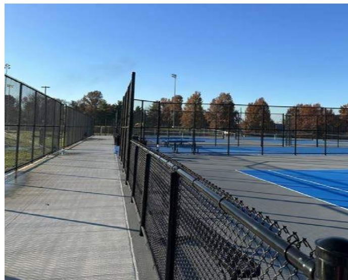
East Concourse Looking South
