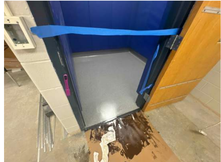
Safe Room with new epoxy floors
