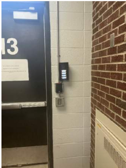
Door 13 low voltage card reader and video intercom installed
