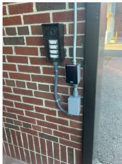
Exterior of Door 13 and video intercom and card reader installed but not fully operational yet
