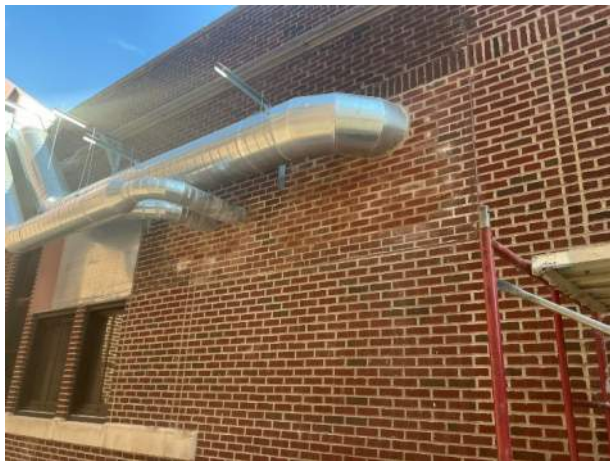
Brick patch at exterior where dust collection enters.
