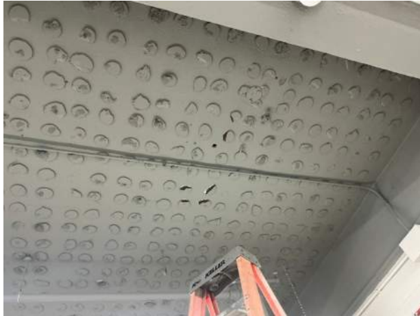
Attempt to remove pucks in the scene shop was unsuccessful, came off in pieces and not easy to remove
