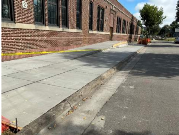
Exterior ramp concrete poured
