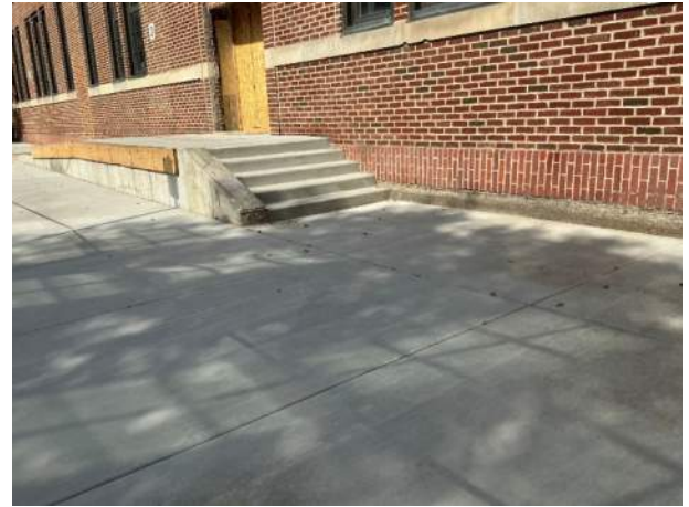
Concrete stoop and steps poured
