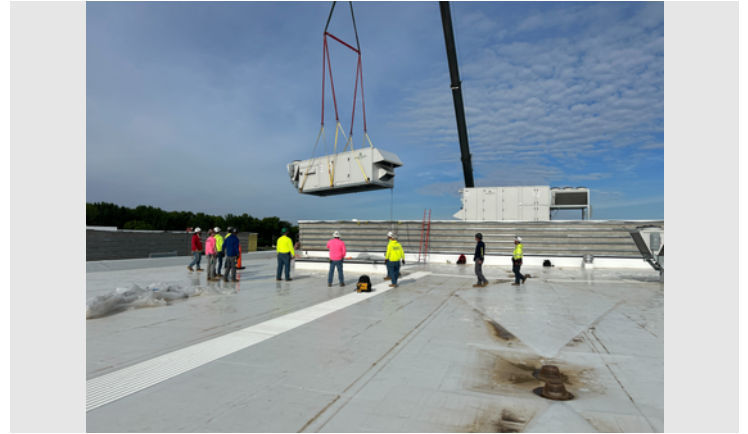
Description: Setting the rooftop unit on the cafeteria
