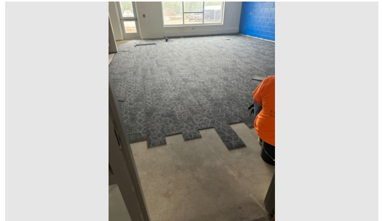
Description: Carpet being installed in a Kindergarten classroom
