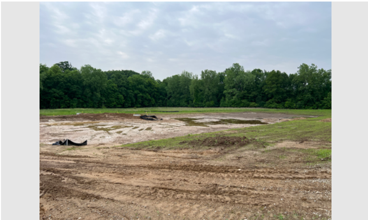
Description: New retention pond on the South East corner of the property.
