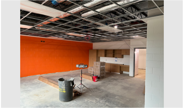
Description: Zone B first floor classroom
