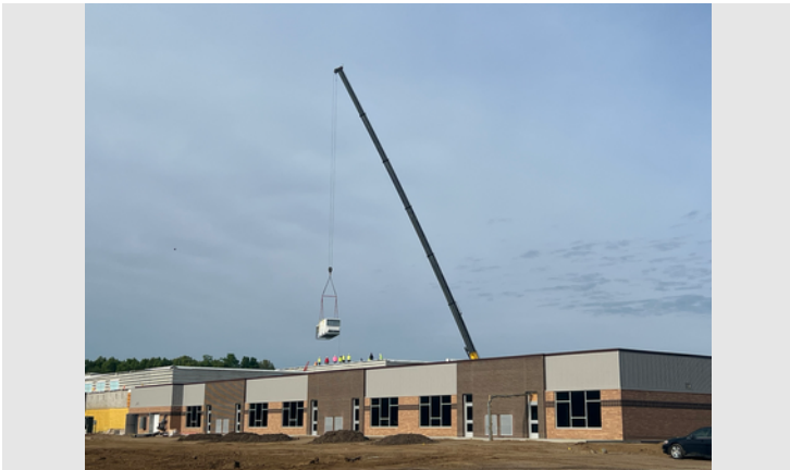
Description: Setting the biggest rooftop unit on the main gym, 10,500 lbs.
