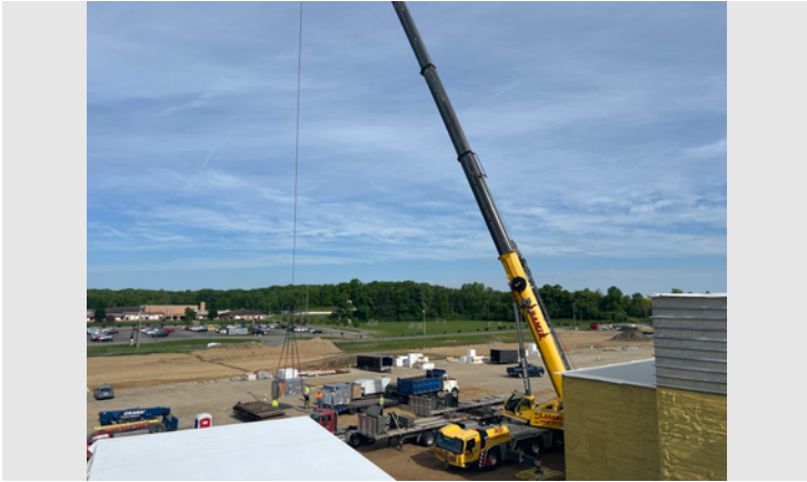
Description: Crane picking rooftop units
