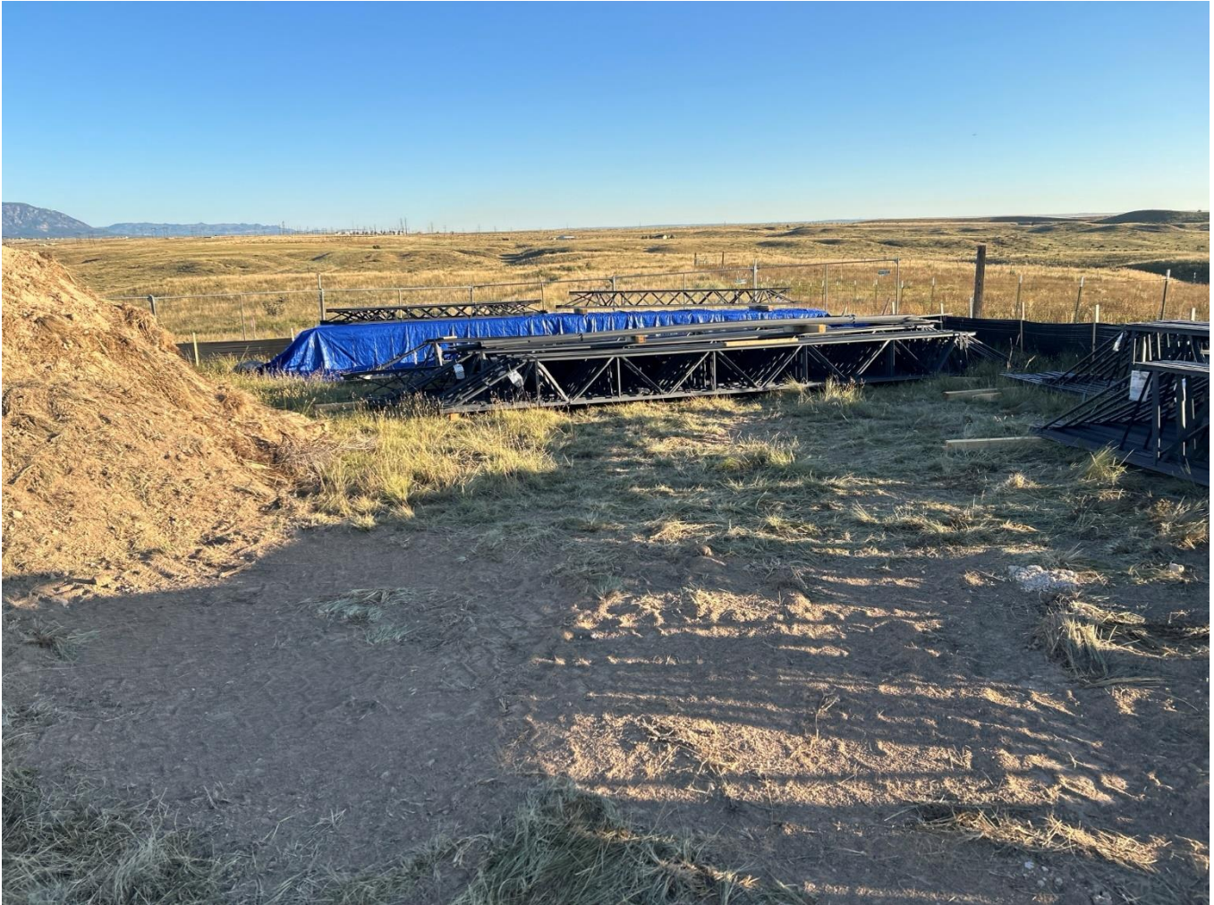
Steel Delivery for New Structure
