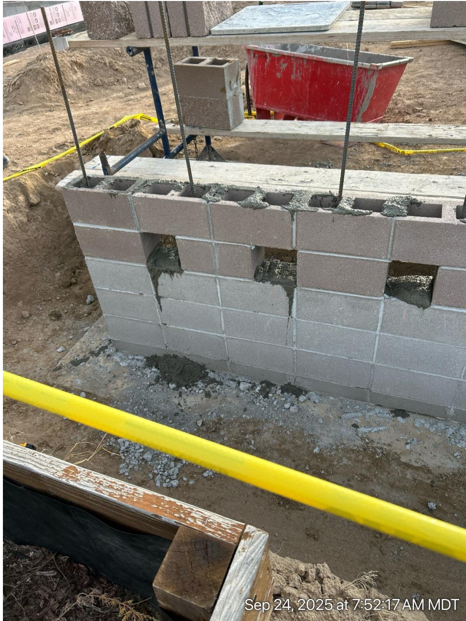
Site Wall Block Fill
