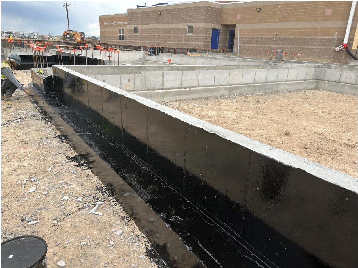
Foundation Sealing
