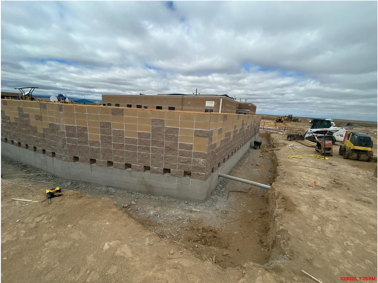
Site Wall Progress
