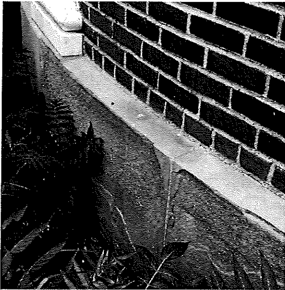
Spalled section at the southeast corner:
