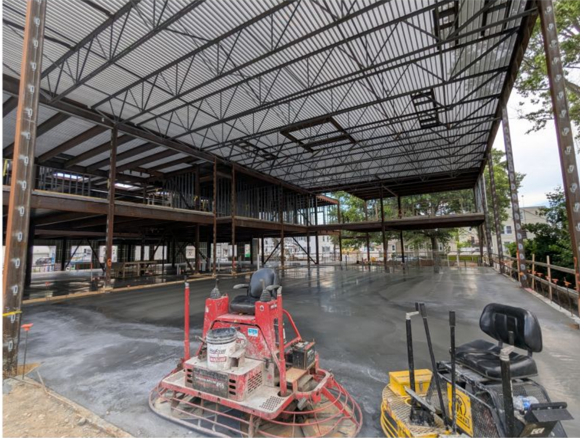
Slab on grade poured – view of Gym/Cafeteria
