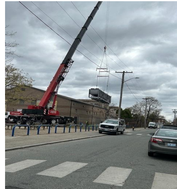
New Lima chiller being installed
