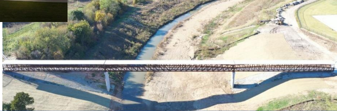
Cheney Hills Bridge (500 foot bridge connecting Haltom City to Richland Hills)
