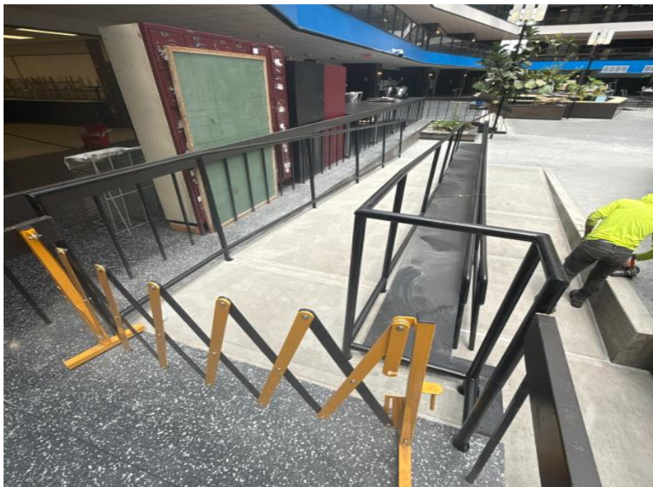
Hempstead HS – Interior Ramp
