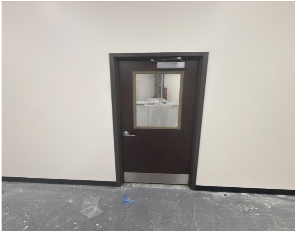
Hempstead HS – C Building Classrooms
