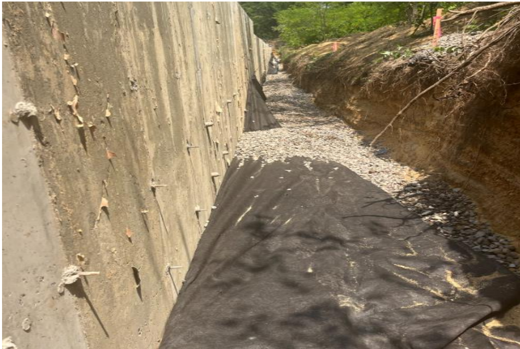
Hempstead HS – Tennis Courts
