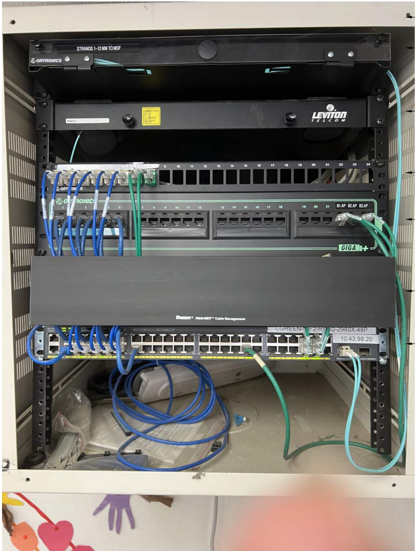
RACK - EXISTING CONDITION
