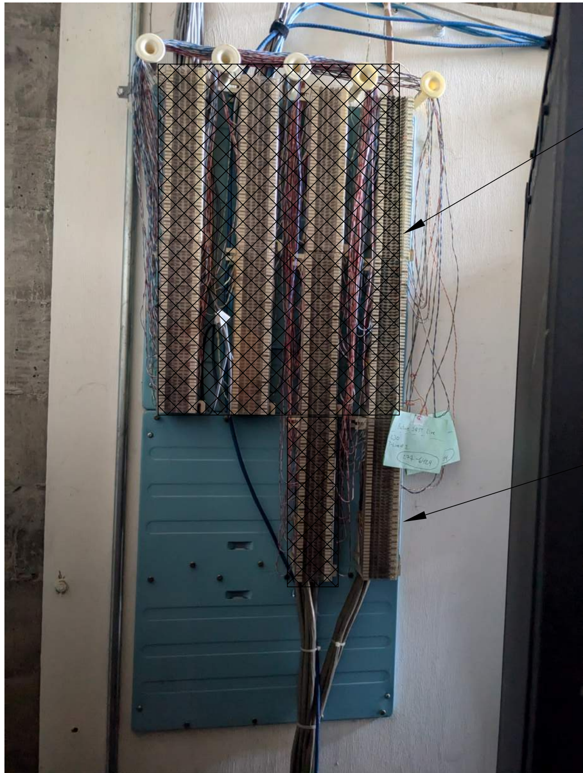
PICTURE DETAIL - 66 BLOCK DEMO
