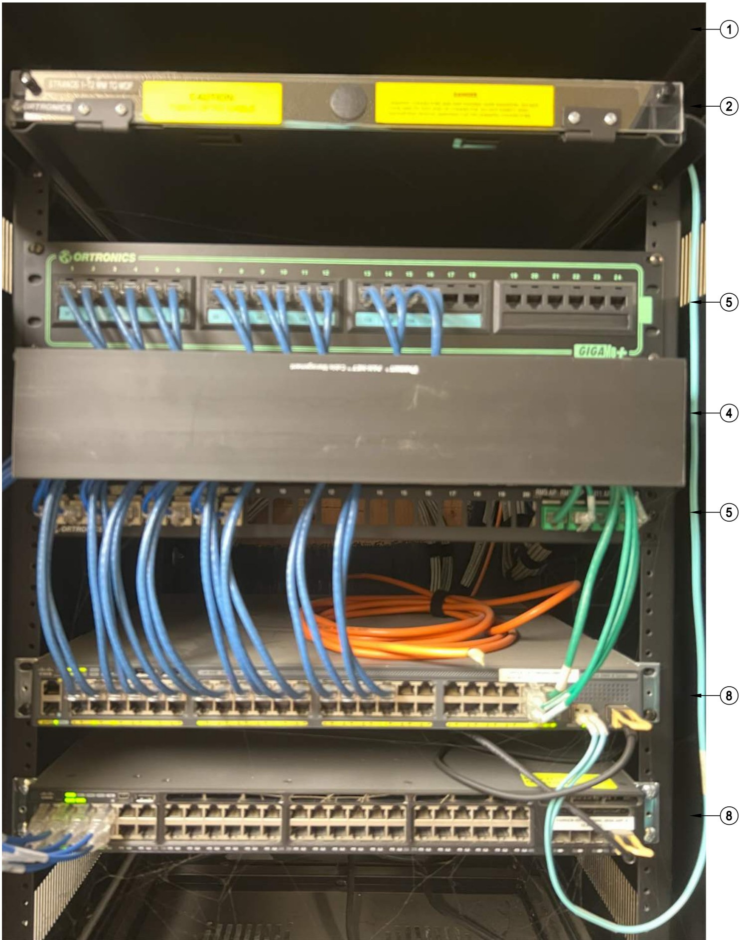
RACK - EXISTING CONDITION
