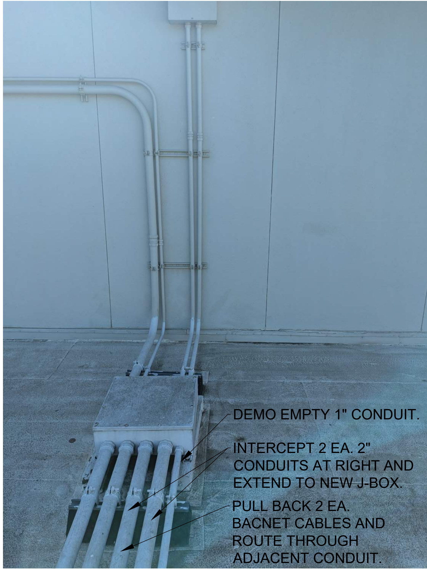
PIC DETAIL - (N) J-BOX AT MP ROOM CANOPY
