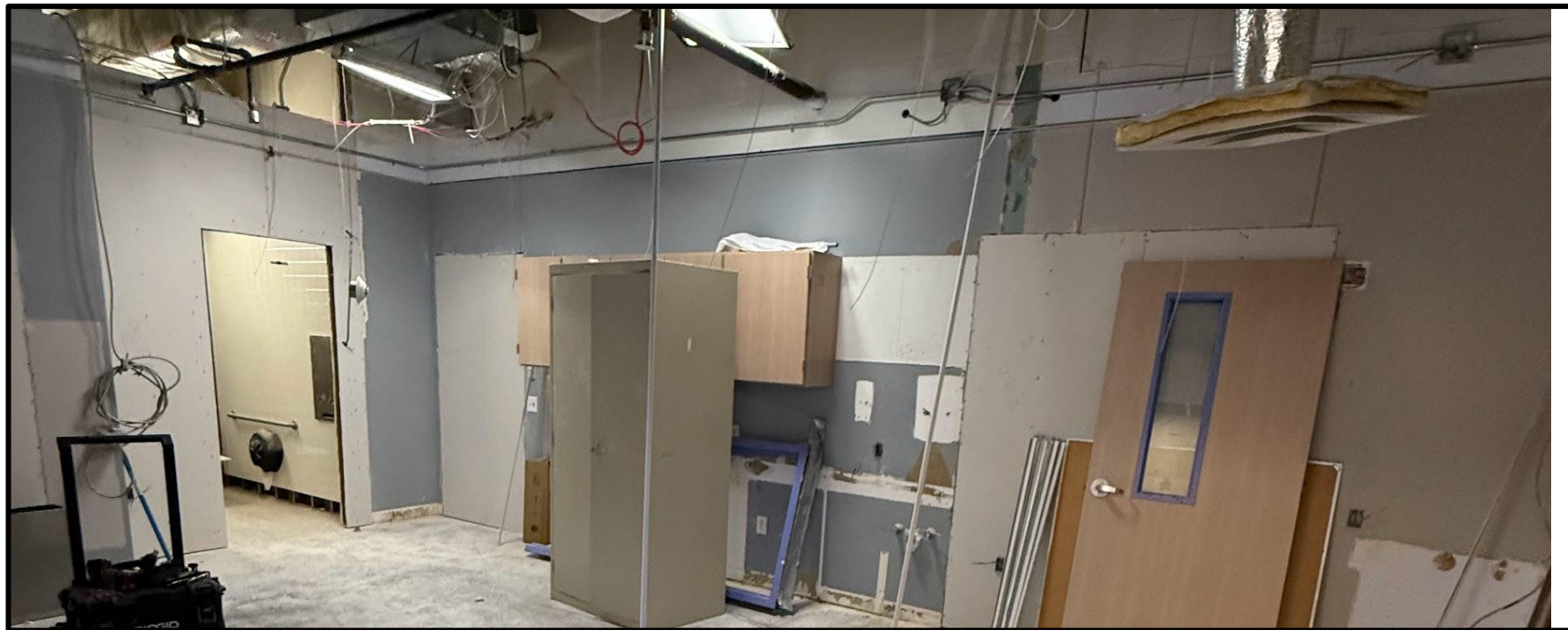
Fields Store Clinic Remodel
