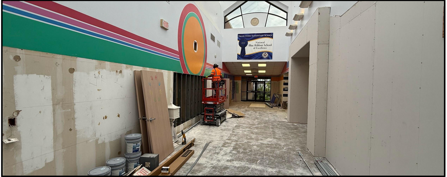
Fields Store Entry Corridor
