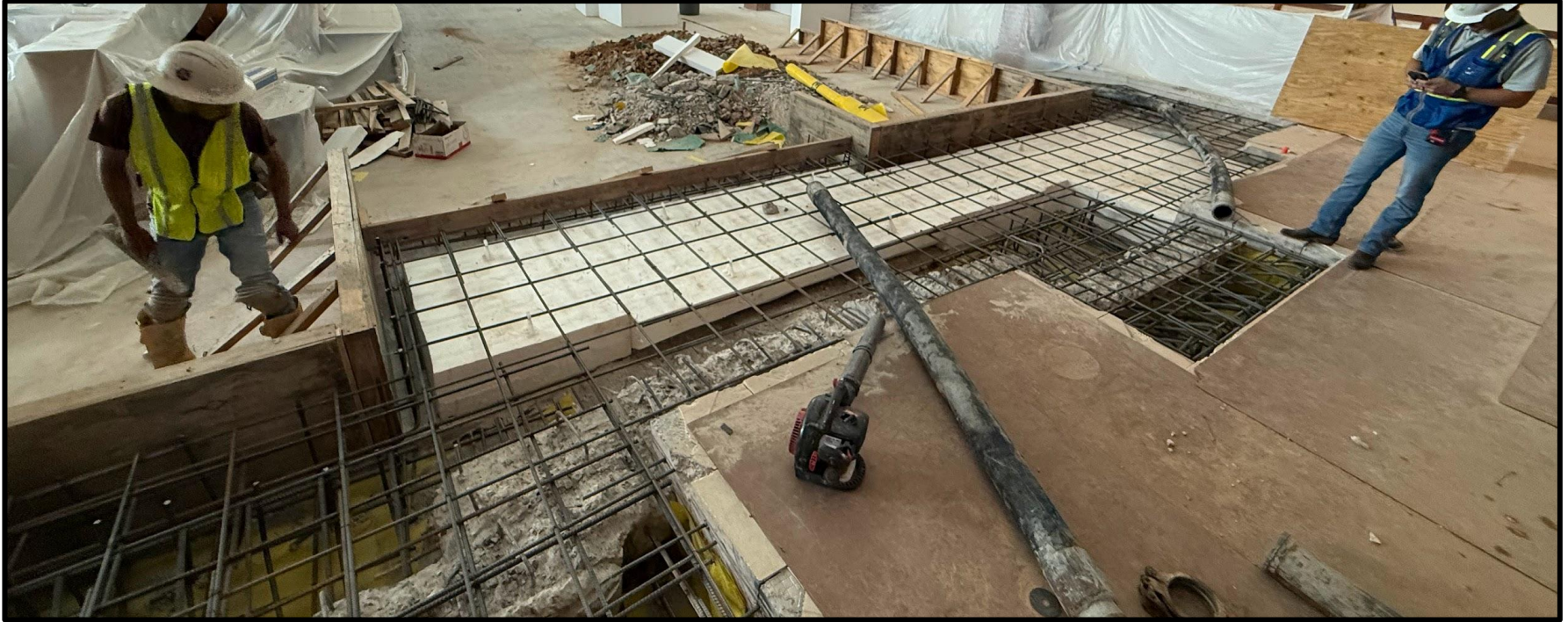
TES Library New Entrance
