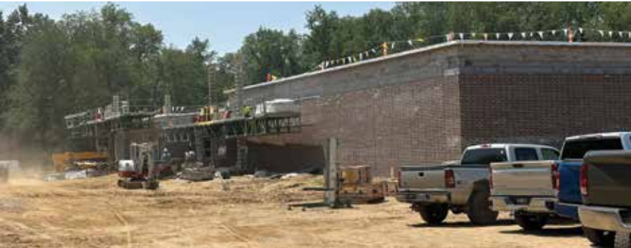
The new district kitchen on the west side of Kalamazoo quickly took shape over the summer.
