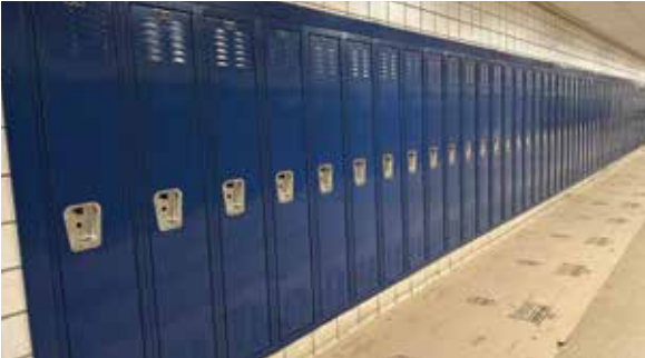
Over the summer, new lockers were installed in the 600 wing of Maple Street Magnet School for the Arts.
