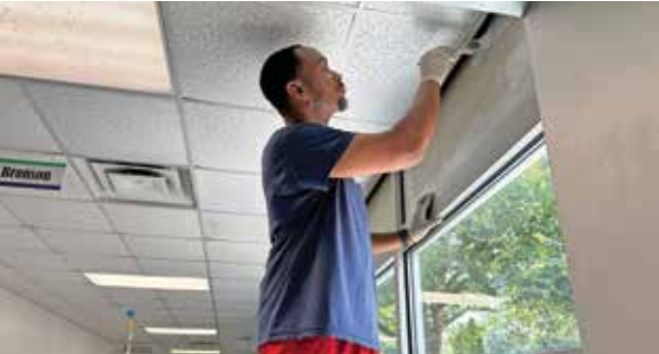
Steven Ray Jr. works on a window panel as part of this year's summer paint crew at Spring Valley Center for Exploration.
