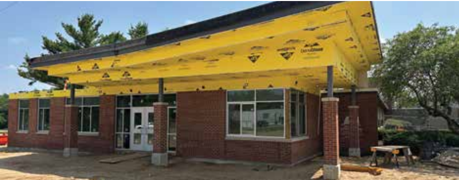
The district's South Westnedge building received several upgrades this summer, including a new secure entrance.
