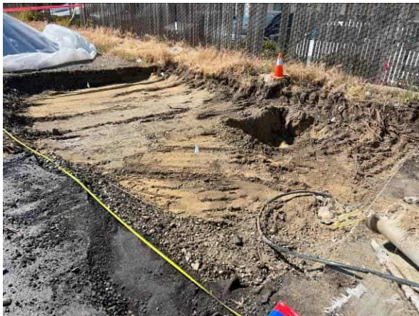
Photo #3 View of excavated area and sample locations.
