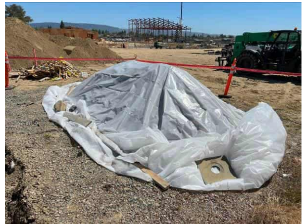
Photo #4 View of generated soil stockpile.
