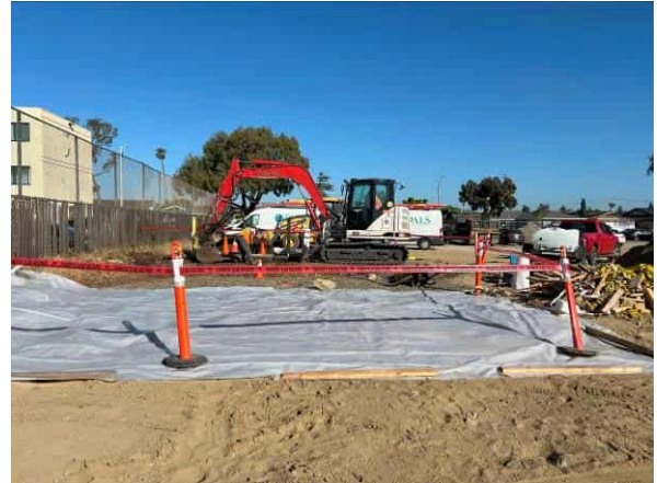
Photo #2 View of soil excavation and soil removal.
