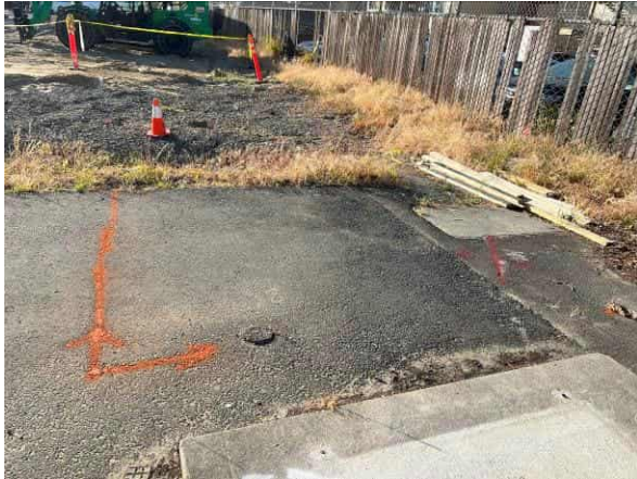
Photo #1 General view of the area prior to excavation.
