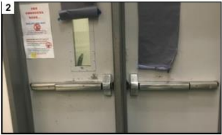
Fine Arts - Replace aged doors and frame.
