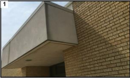
Replace metal soffit trim and wood blocking, typical. Acid wash plaster and masonry veneer.
