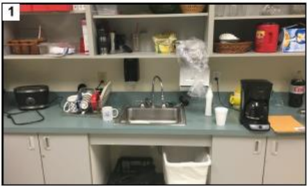
Admin - Replace aged casework in lounge.
