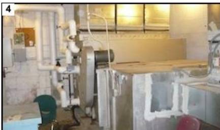
Trane 3 zone multi-zone air handling unit
