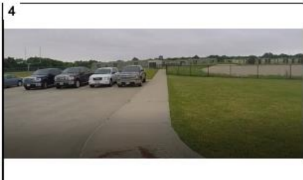
No accessible route to football field or track.
