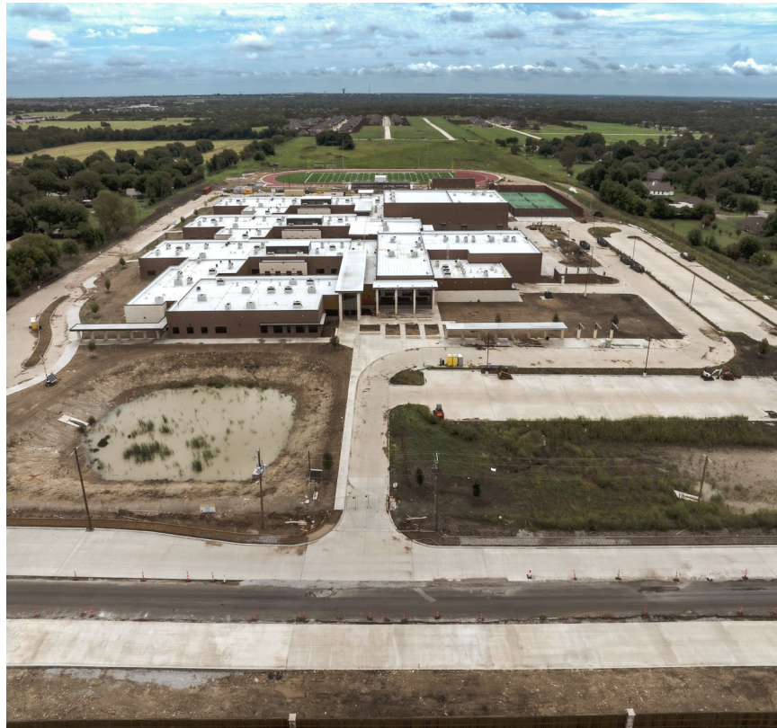
Arial view of the new Shaw Middle School construction in June 2025
