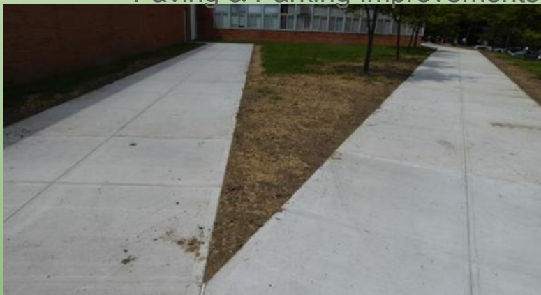
Paving & Parking Improvements
