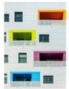
John Roman Architects - Independence Library and Apartments, Chicago, IL. Photo by James Ford.
