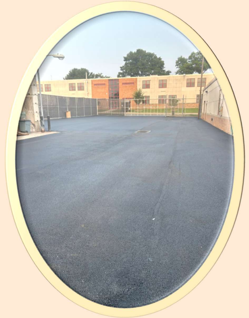
Maintenance Shop Lot
