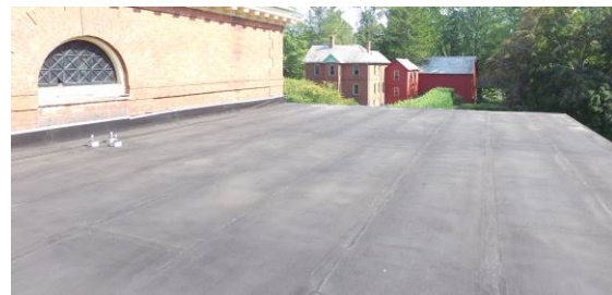
View from West to East
