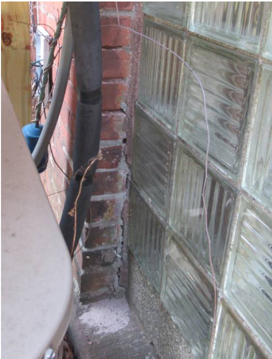
Mortar deterioration
