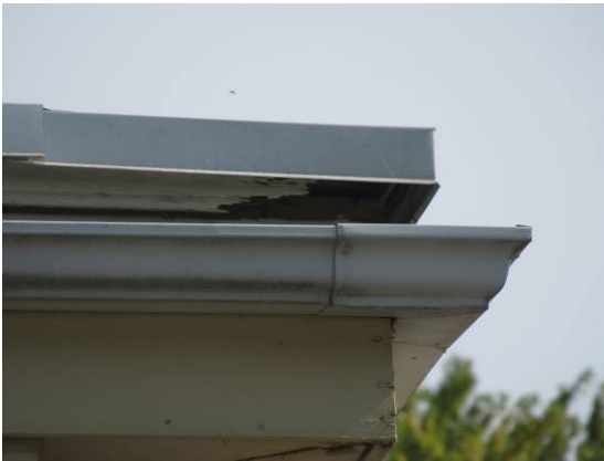
Repair/replace rotted woodwork.
