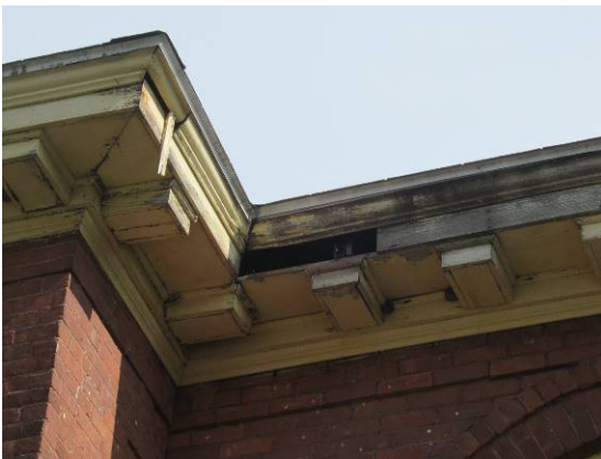
Repair/replace rotted woodwork.
