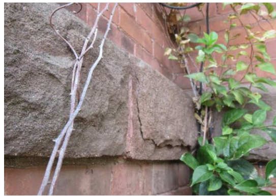
Stone spalling/deterioration
