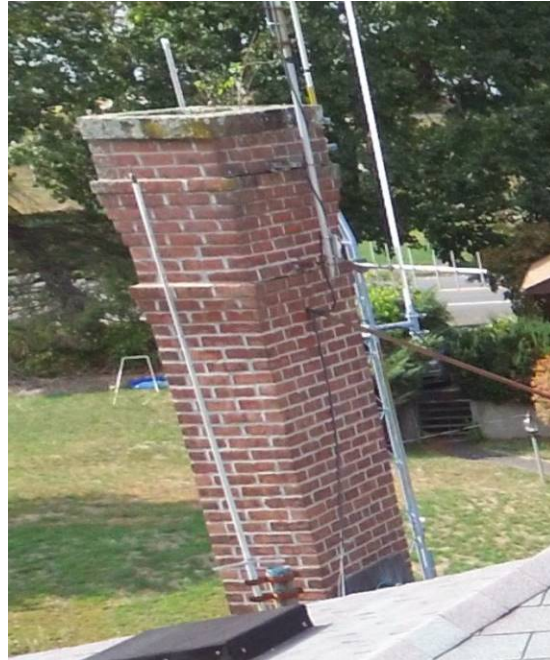
Review chimneys for repointing (Being used for support of antennas)
