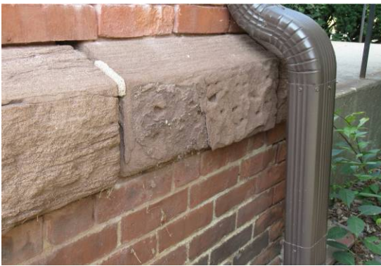
Stone spalling/deterioration
