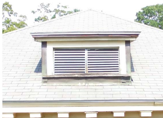
Dormer Elevation (Repair Flashing)
