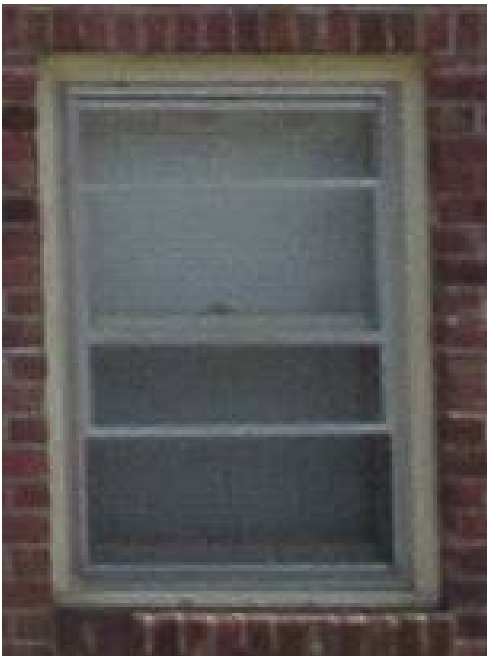
(4-Units, 2 with security bars) – 1960 Building
