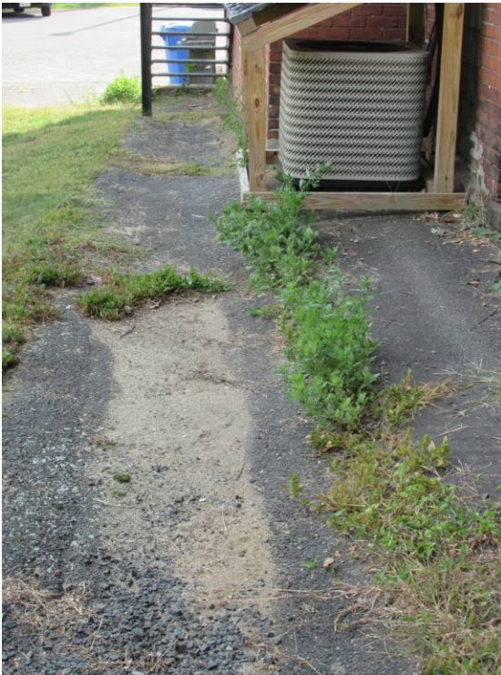
Paving added along the perimeter of the building (East Side)
