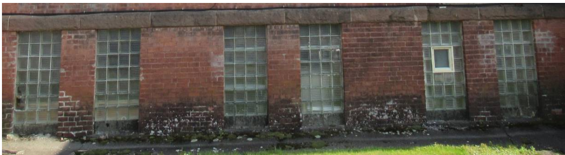
(6-Unit, 5 same, 1 custom) (This photo is from west elevation, the east is similar but has too many obstructions for a single photograph.)
