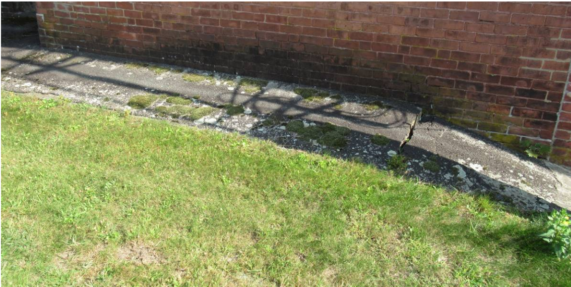
Paving added along the perimeter of the building (West Side)
