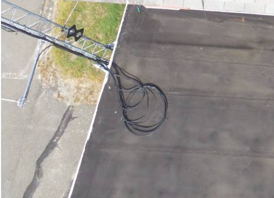
Coiled cable (Provide roofing mat or additional layer of roofing below cable for a wear layer.)
