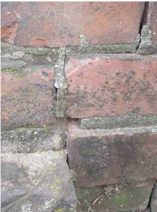
Mortar deterioration
