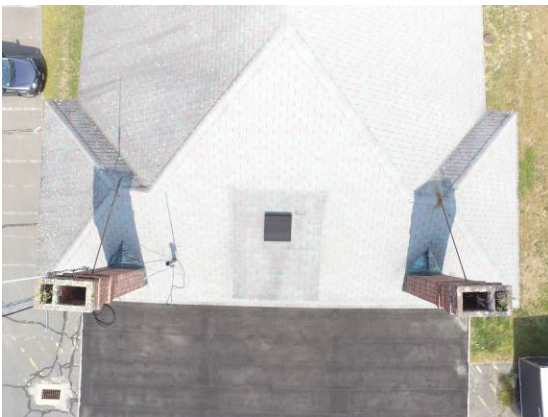
South Chimneys – vegetation, support (Examine cricket and flashing behind each chimney.)
