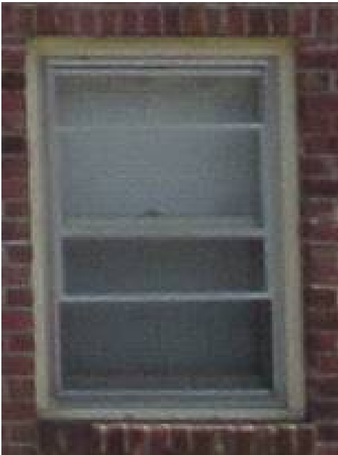
(6-Units, 2 with security bars) – 1960 Building
