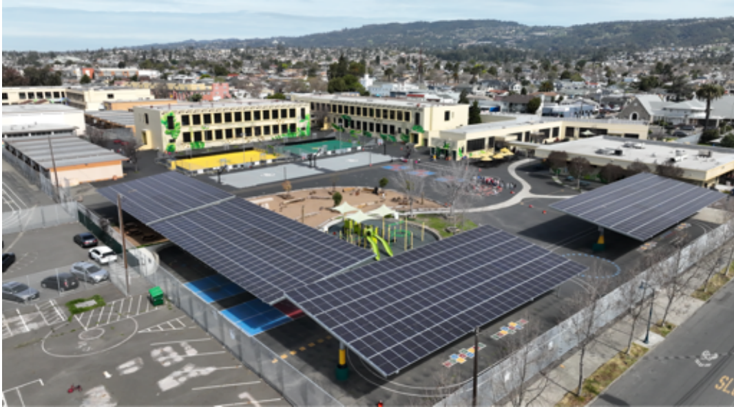
Photo: Solar Project at Lockwood Steam Academy
