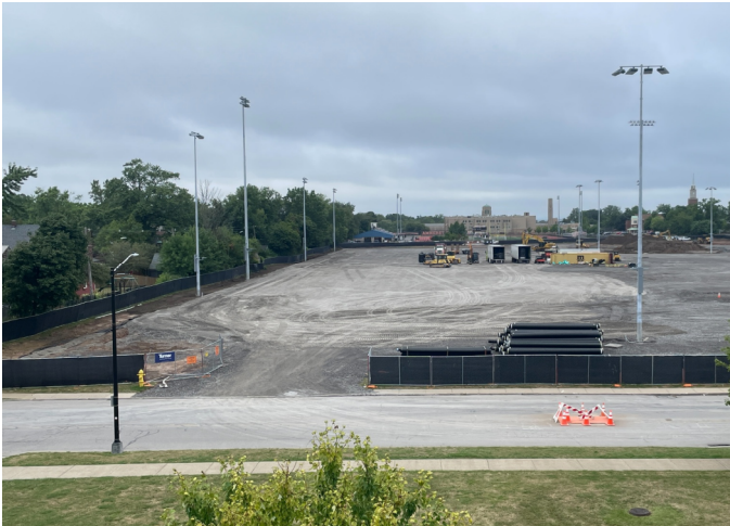
Turf Complex - Athletic Lighting Installation
