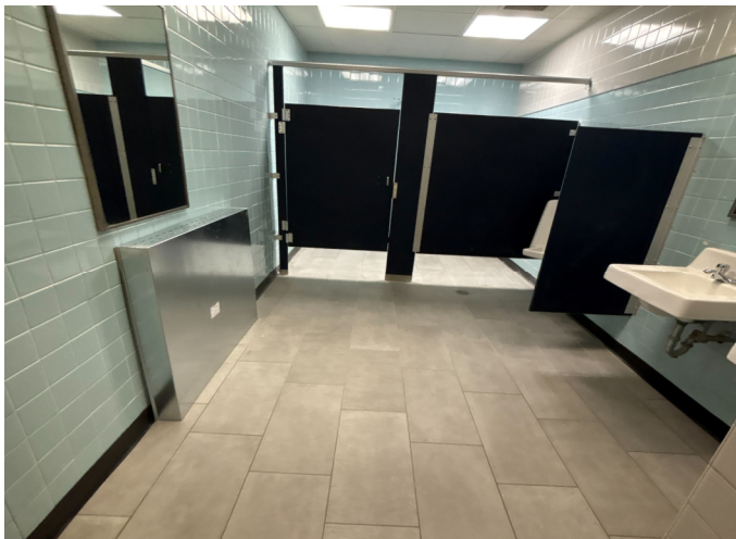
SW - Boy's Bathroom New Floor Tile
