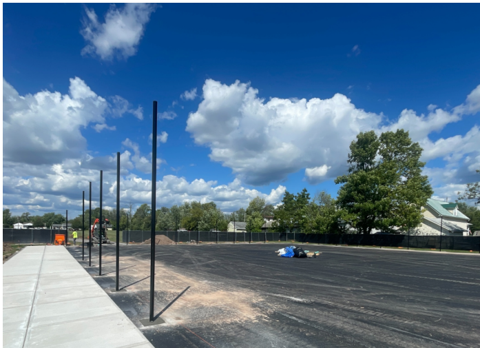
Windermere Tennis Courts - Binder Pavement + Fence Pole Installation
