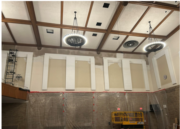
High School - Auditorium Plaster Restoration
