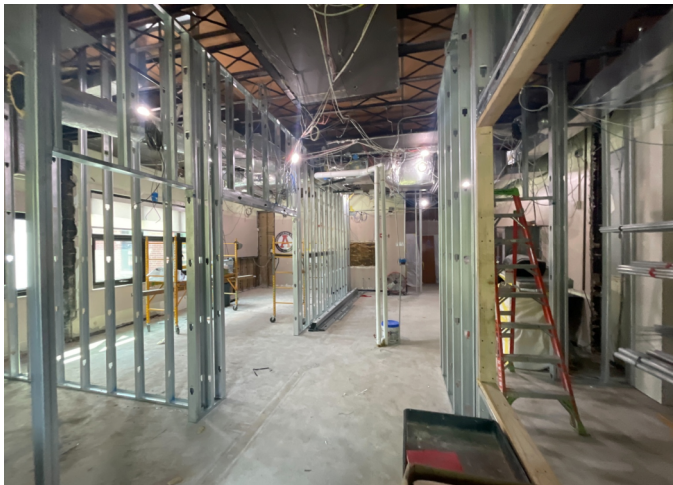
SW - Main Office Metal Framing
