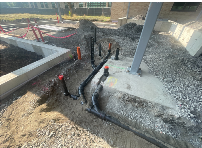
New UPK Addition - Underslab Piping
