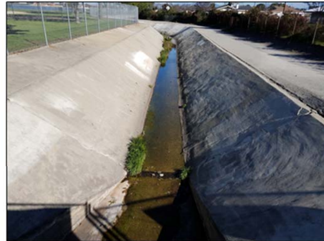
PHOTO 4: View looking north of the Palos Verdes Lateral Storm Channel in the east project site boundary.
