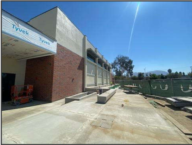
New Gym Building - Lobby entry, concrete stairs, and walkway
