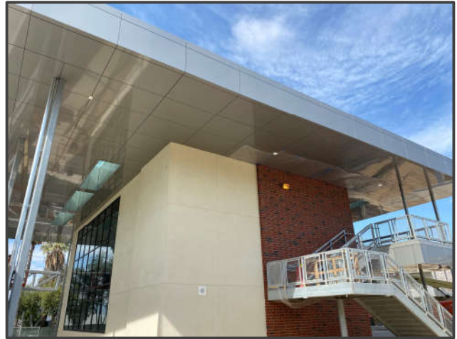
New 2-Story Science Classroom Building - Brick veneer sealer prep work
