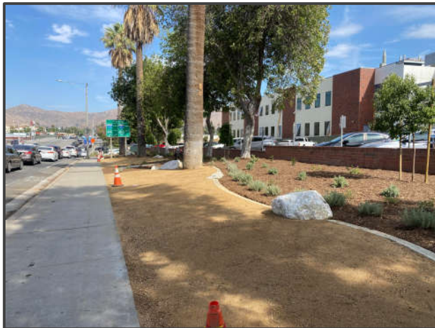
New 2-Story Science Classroom Building – Front landscaping work
