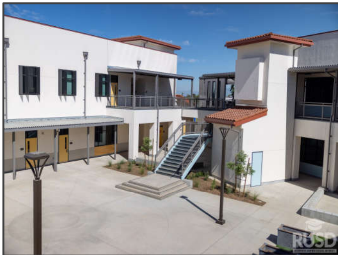
Building F - Quad Area
