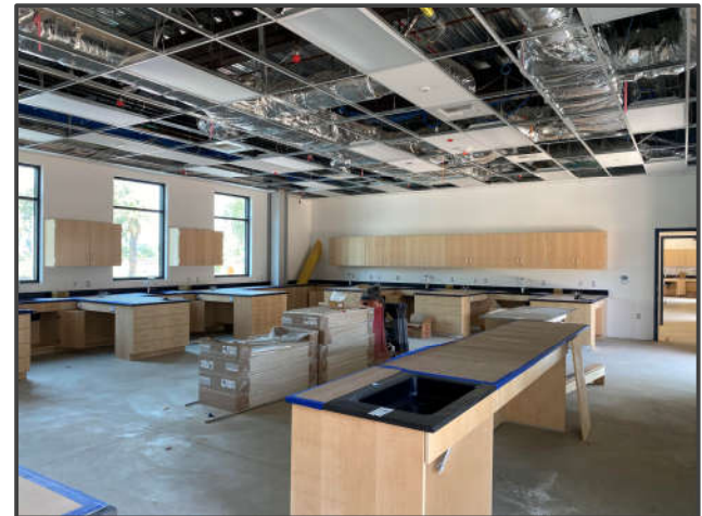
New 2-Story Science Classroom Building - Lab classroom sink installation work
