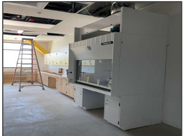
New 2-Story Science Classroom Building – Fume hood installation work
