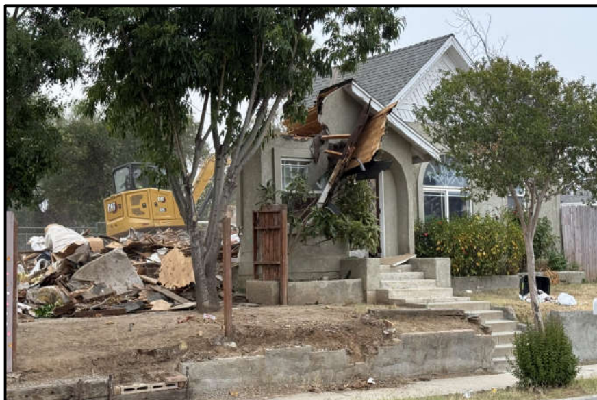
Eastside – Demolition of residential structure
